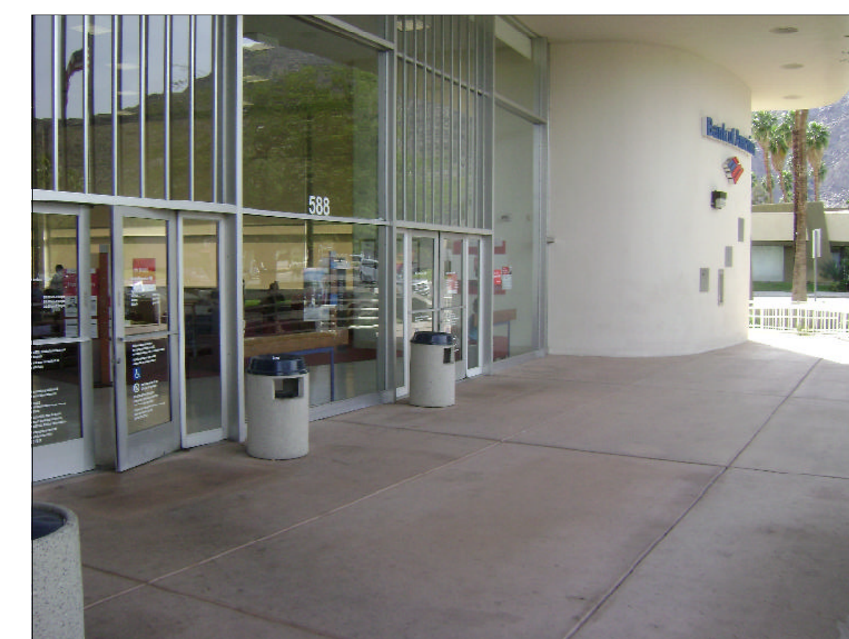
VIEW OF ENTRY
