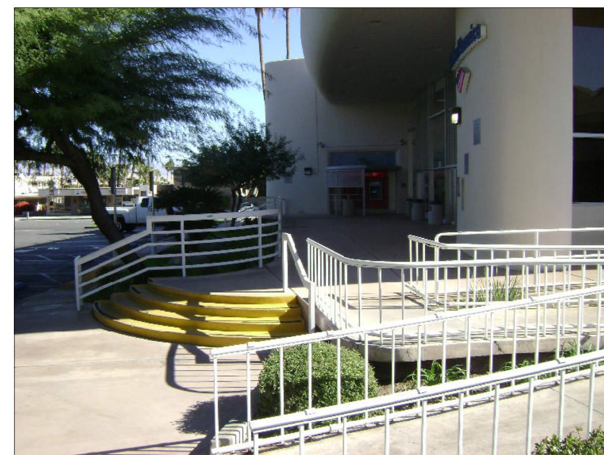
VIEW OF EXISTING RAMP
