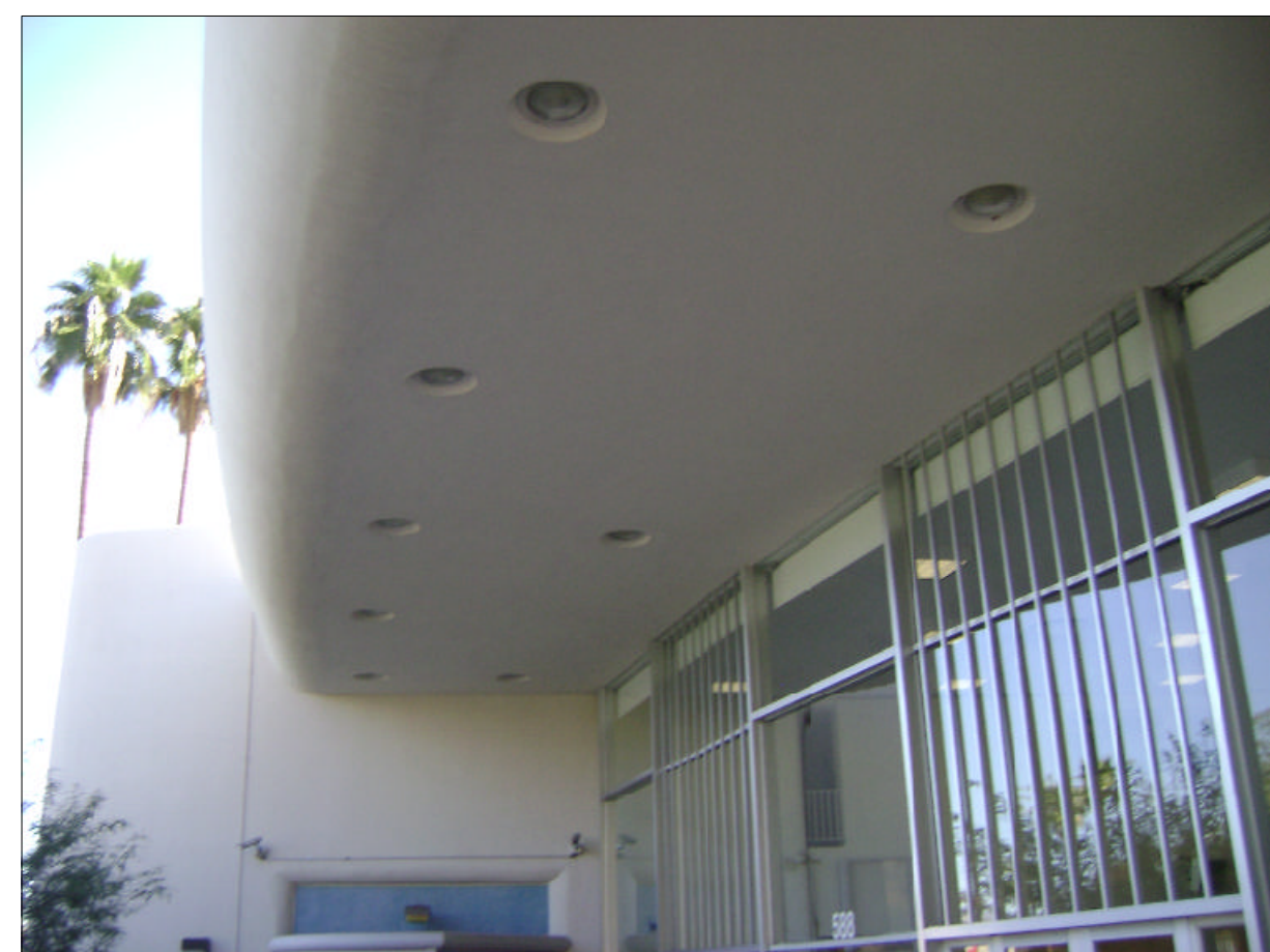
VIEW OF SOFFIT
