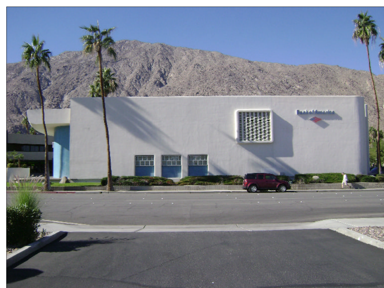
VIEW OF WEST OF BANK
