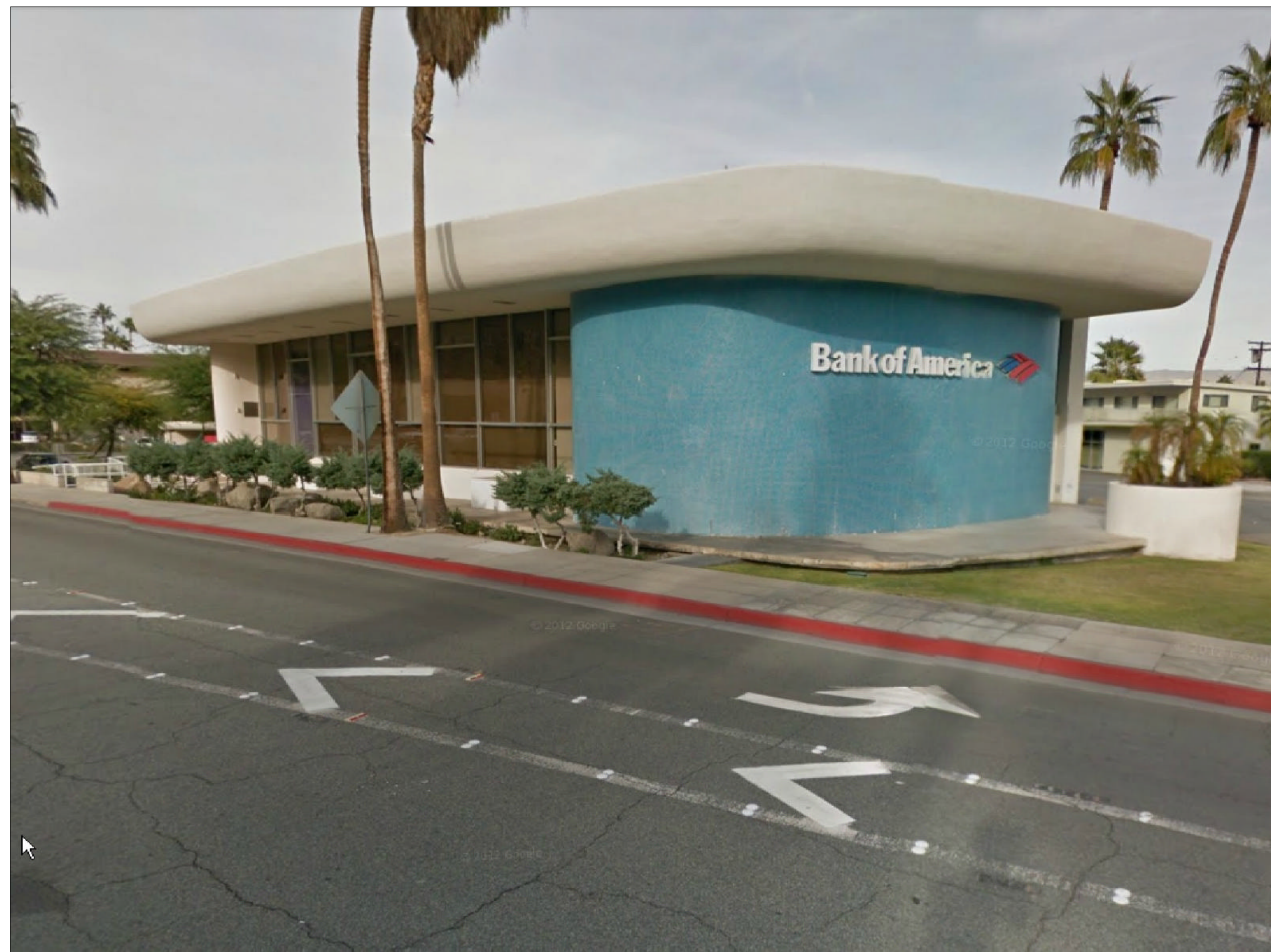
VIEW NORTH-EAST OF BANKING CENTER
