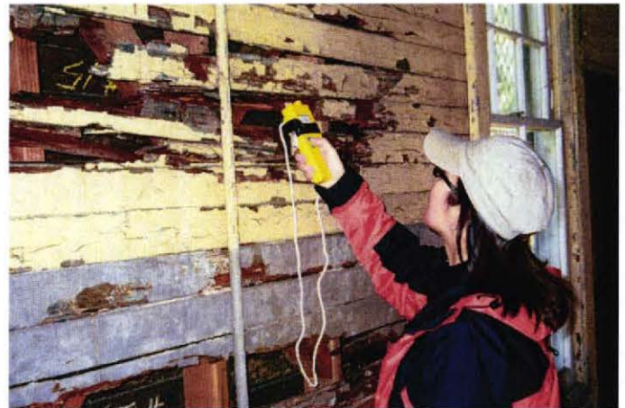
Measuring Moisture at Wood Decay
