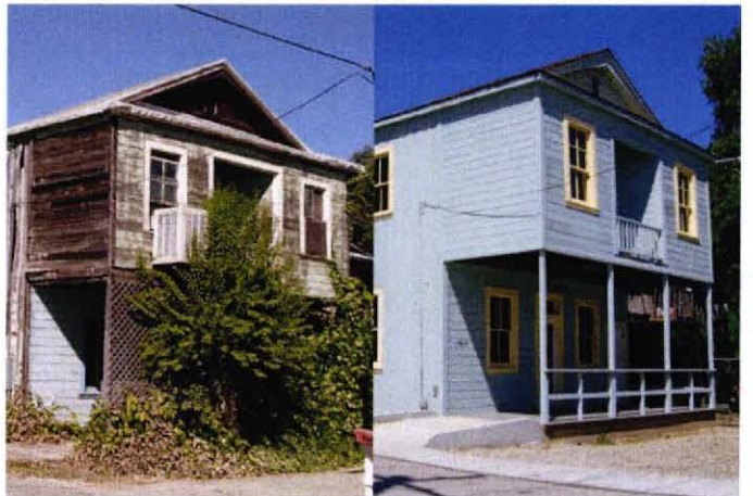
Locke Boarding House
