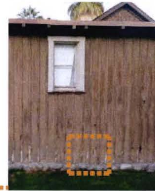
VERTICAL BOARD & BATTEN OVER STUD FRAMING
