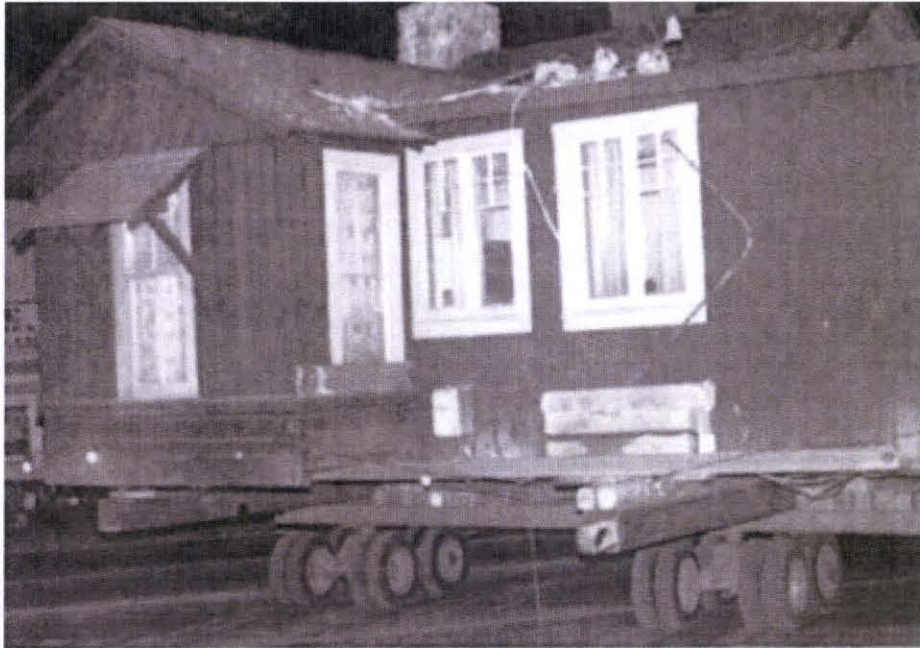
MOVING THE CORNELIA WHITE HOUSE IN 1979 TO THE VILLAGE GREEN PARK
