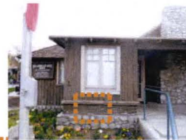
VERTICAL RAILROAD TIES WITH BATTEN ABOVE SHAPED WATERTABLE OVER HORIZONTAL RAILROAD TIES
