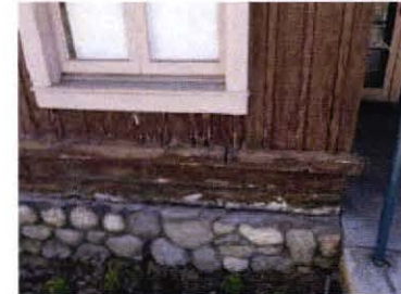
WATER DAMAGE TO RAILROAD TIES & WATERTABLE
