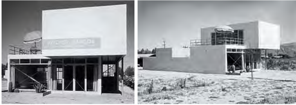
Kocher-Samson Building (1934, Kocher and Frey; HSPB-79). Source: Palm Springs Life , Desert Treasures Gallery.
