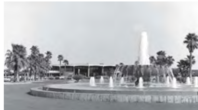
Palm Springs Airport fountain, c. 1970s. The famous fountain was designed by renowned Mexican architect Julio de la Pena as a gift to the city, and was constructed from stones brought in from Guadalajara. In 2009, it was named in honor of the City's iconic former Mayor Frank Bogert. (PHS)
