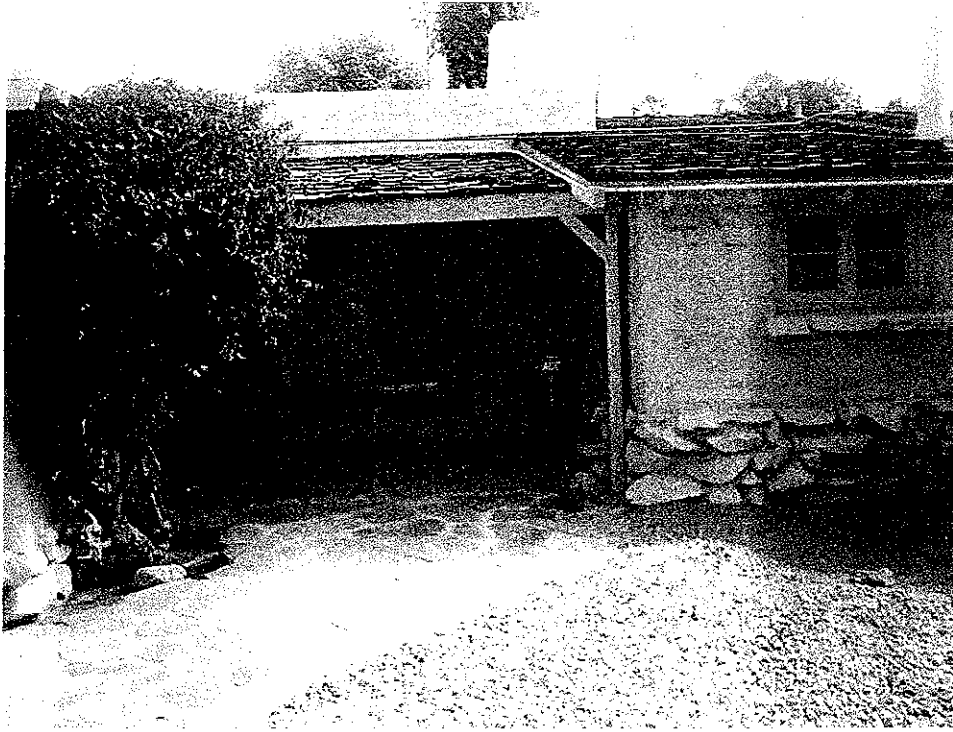
The side porch presents examples of Casablanca Adobe's varying roof styles, its rock foundation, a deep cut-stone window sill, and scenes of decorative tile.
