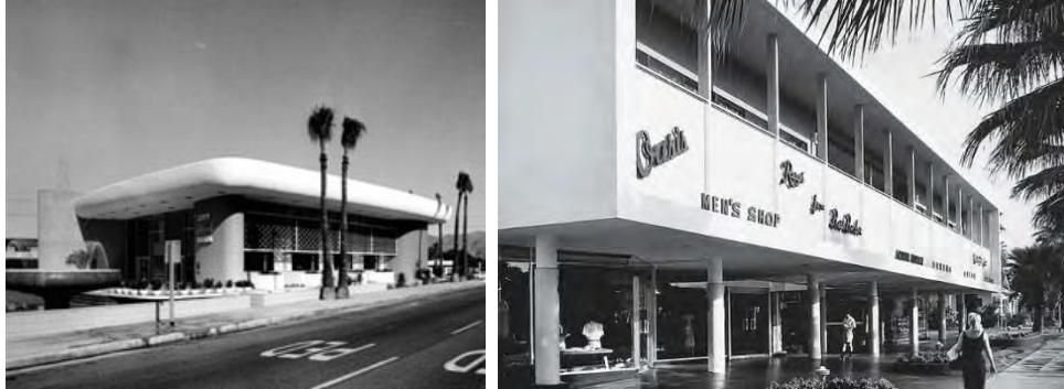
L: City National Bank (1959, Victor Gruen Associates). Source: Bill Anderson/Courtesy Palm Springs Historical Society via Palm Springs Life Archives. R: The Oasis Building (1952, Williams, Williams & Williams). Source: Palm Springs Historical Society as published in Palm Springs Life , "Modern, Naturally."
