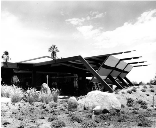
The Springs restaurant (1957, William Cody; demolished). Source: Lost Palm Springs.
