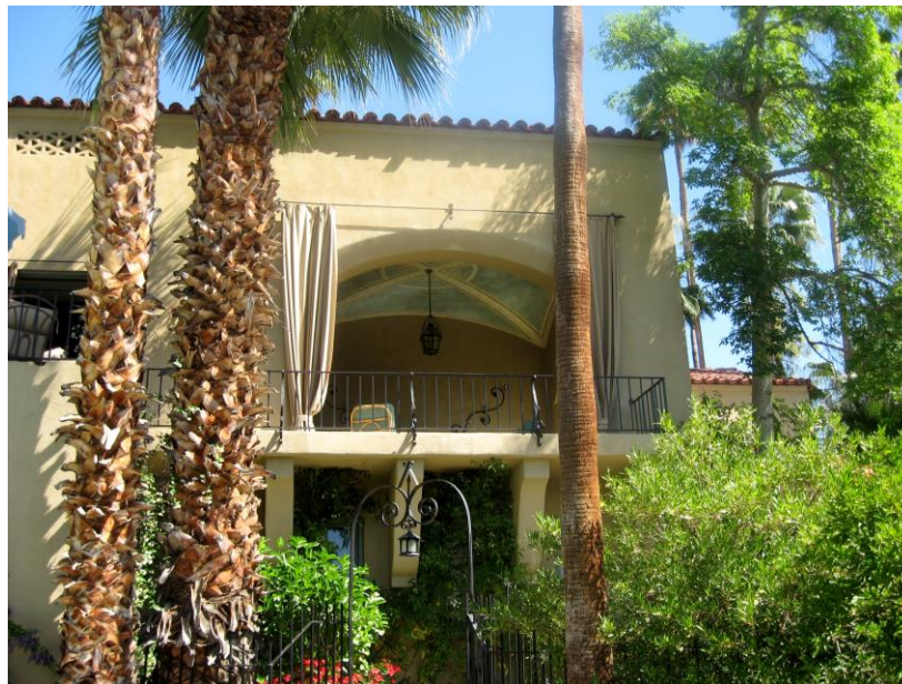
A view of the Bishop House showing the decorative corbels used as support for the living room balcony. (Author Photo. May 2019)
