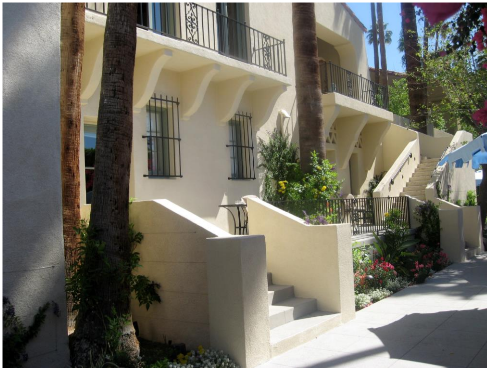
The creation of two ground floor guest rooms required the addition of a small terrace which runs along the center of the southern façade. Staircase on the right is original. (Author Photo. May 2019)
