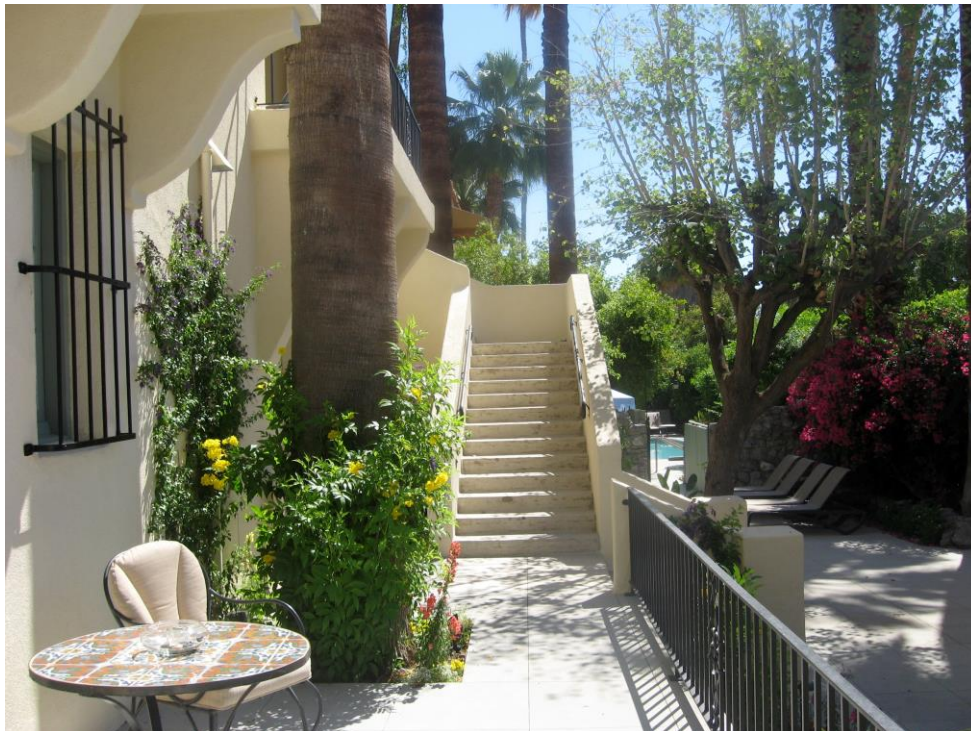
View east across new terrace to original staircase. (Author Photo. May 2019)
