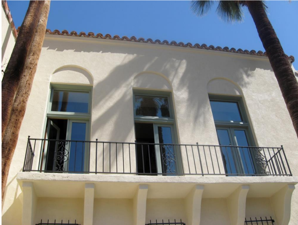
Looking up towards tri-partite French doors opening from living room to balcony. (Author Photo. May 2019)
