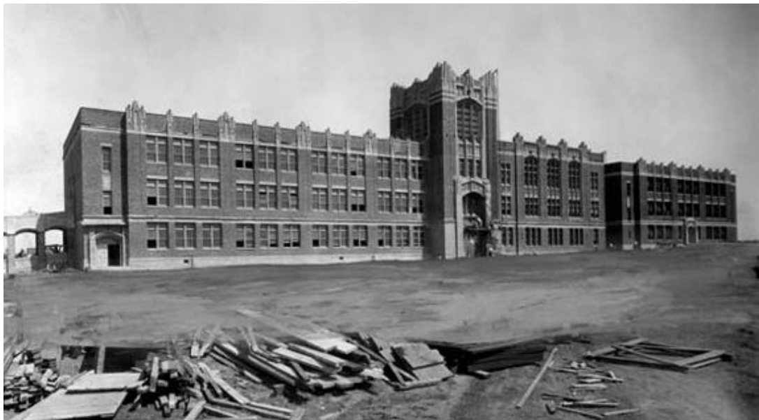
George Washington High School, Los Angeles. (Courtesy Water & Power Associates)
