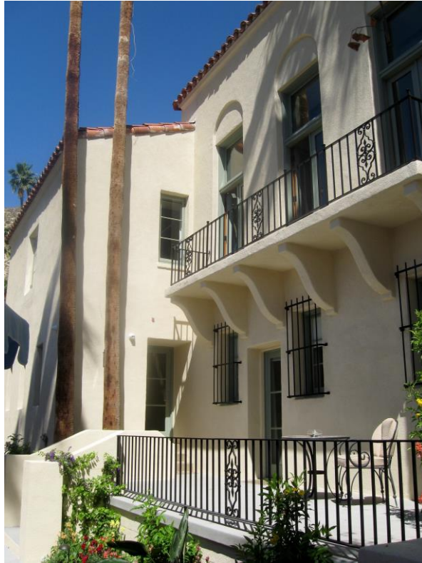
A view of the Bishop House showing the decorative corbels used as support for the living room balcony. (Author Photo. May 2019)
