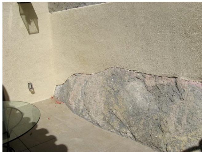
The Bishop House was built as much as possible directly onto the natural topography. (Author Photo. May 2019)
