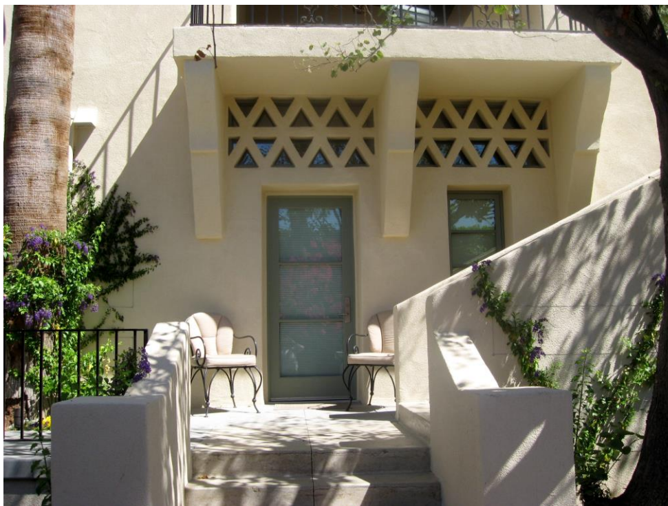
A new door and window were added for the creation of the Orchid Tree guest room. Both window and door were designed to match originals elsewhere on the façade. Note the original artistic vents, which have been glassed in and now provide light to the room. (Author Photo. May 2019)
