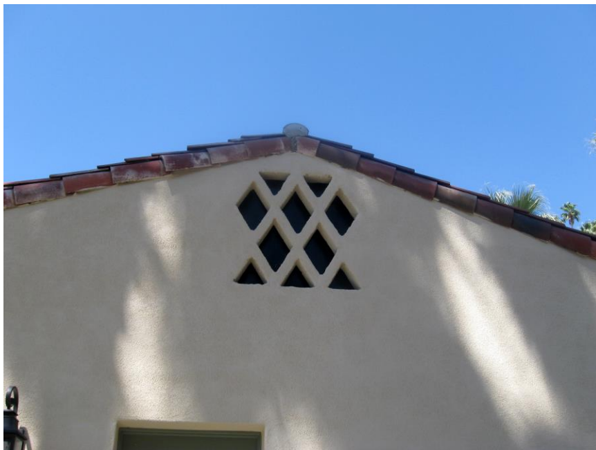
One of the decorative air vents on the Bishop House. (Author Photo. May 2019)
