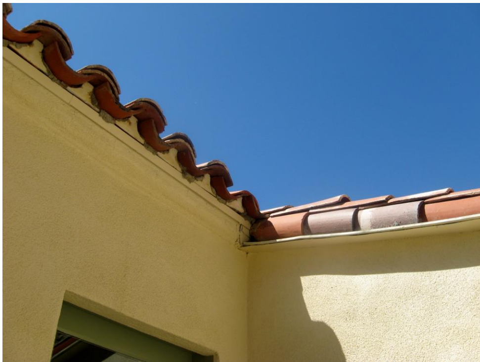
Detail of intersecting rooflines. (Author Photo. May 2019)
