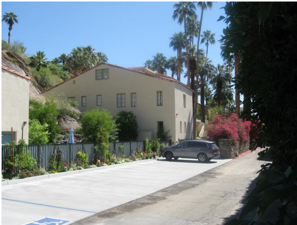
View looking east down Tahquitz Canyon Way. Former garage (now Casita) at left. Current owners were able to create 9 parking spaces and an enclosed private garden terrace. (Author Photo. May 2019)
