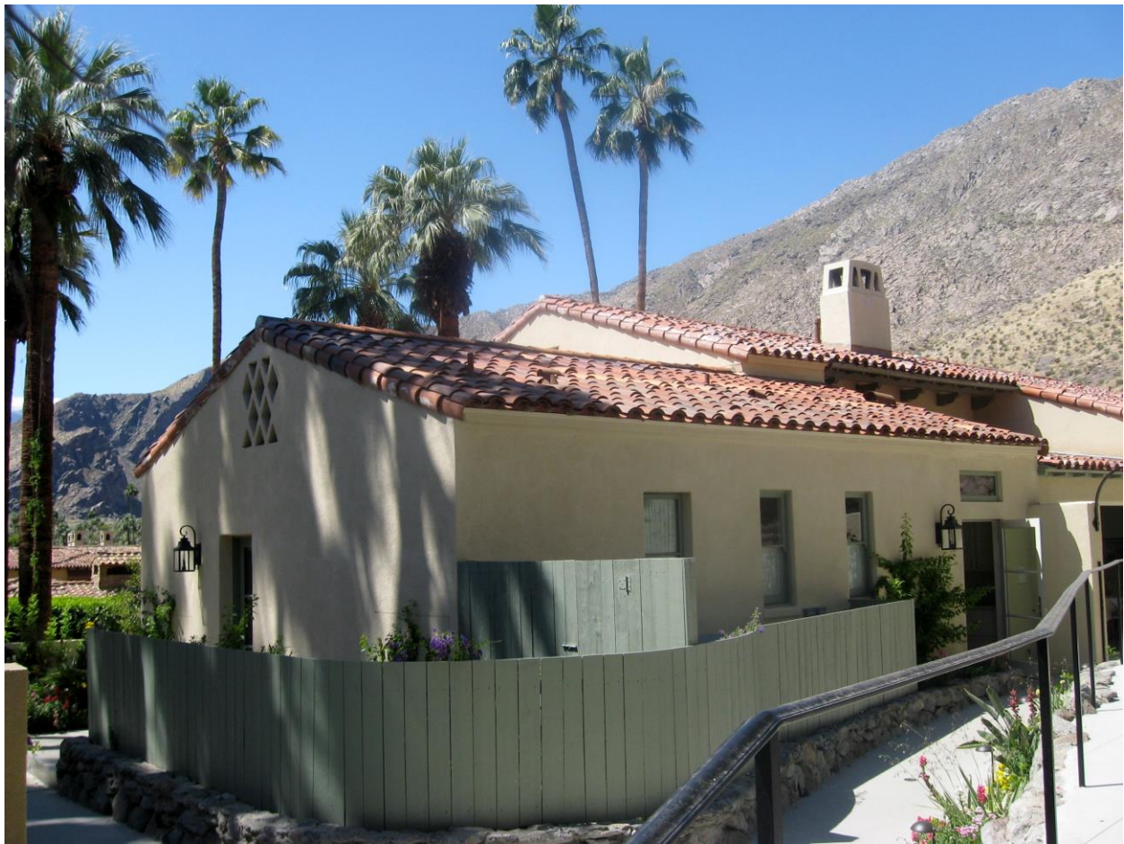
A portion of the north façade, showing kitchen door addition as well as placement of HVAC units as hidden behind wooden fencing. (Author Photo. May 2019)
