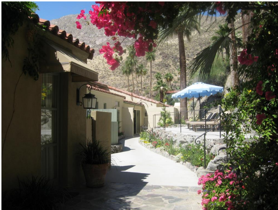
View looking west showing reopened passage between Willows and Bishop House. Note elevated patio on right added during 2017/2018 renovation. (Author Photo. May 2019)
