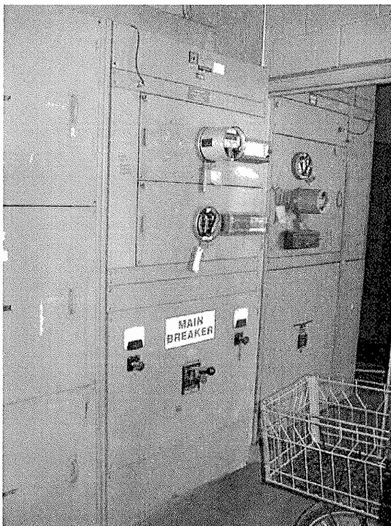
**Figure 7 – Main Service Switchboard at Maintenance Building**
