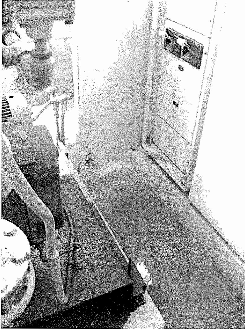
**Figure 4 – Headworks Motor Control Center Door Interference**
