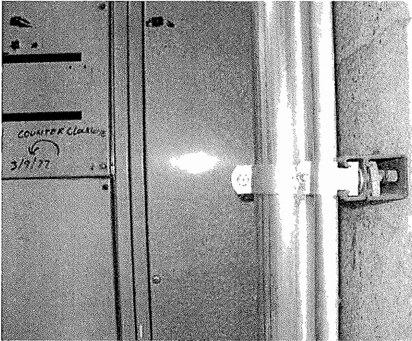
Figure 2 – Switchboard Front Access Interference in Administration Bldg.
