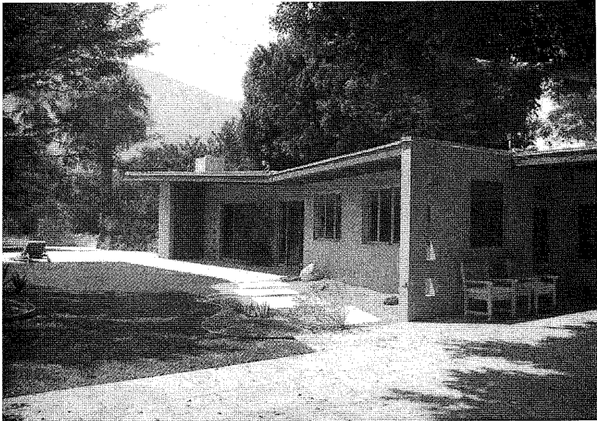
Figure 1 Hugh Stephens Residence, 645 Morongo Road
