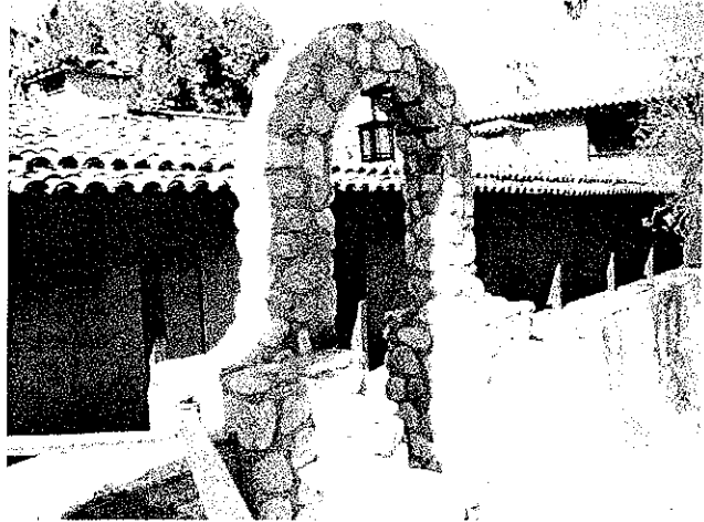
Craftsman stone arch (Label A) house destroyed by fire
