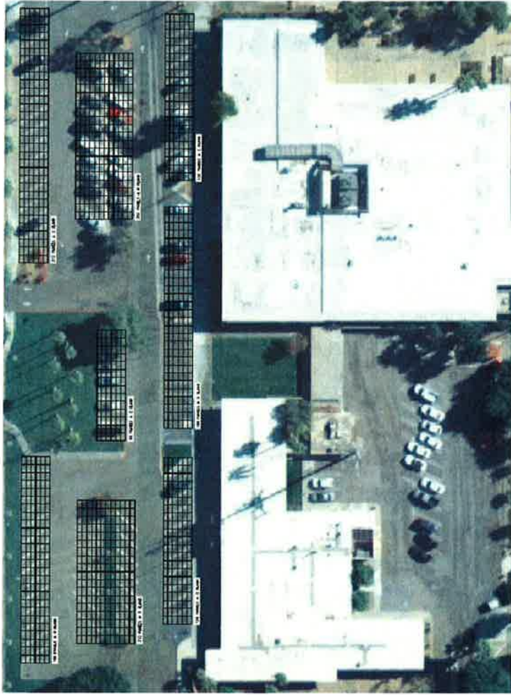
North Lot Carports
