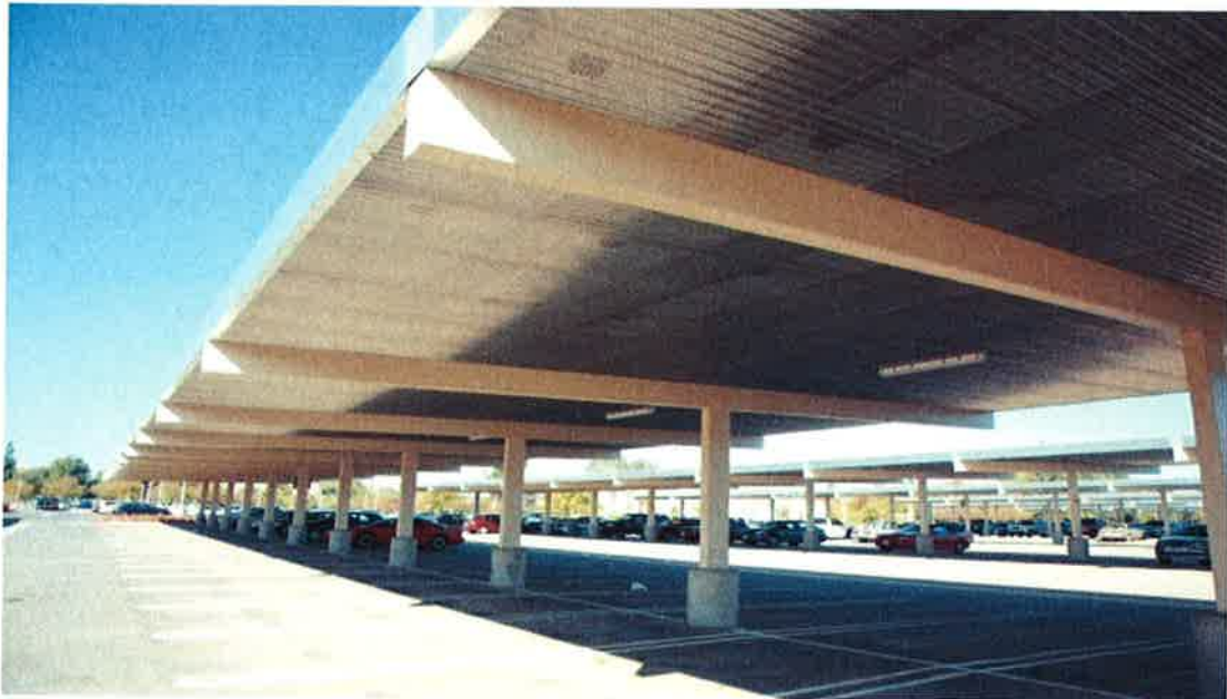
Solar Carport Installation
