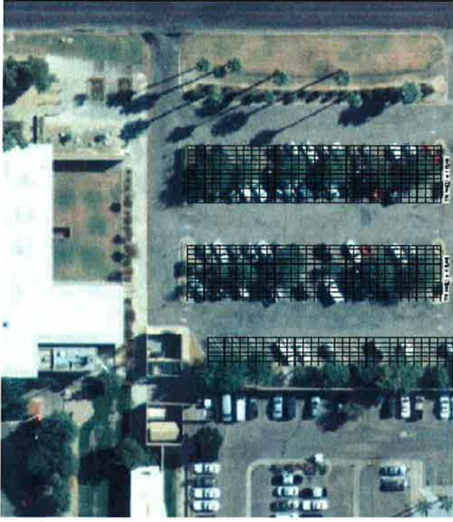
South Lot Carports
