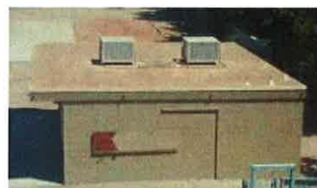
Stadium Concession Stand
