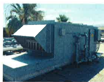
Outdoor Indirect Evap Cooler
