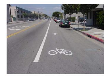
Figure 3: Bike Lane Striping and Stencil
