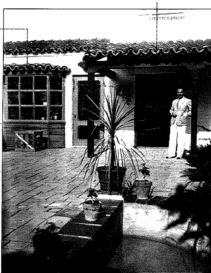
3. HISTORICAL PHOTO AT COURTYARD LOOKING NORTH
