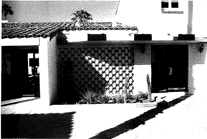
Existing block wall and screen to be removed
