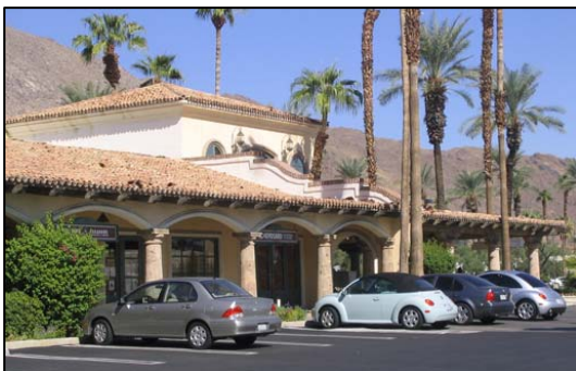
Interesting architectural detailing, large display windows, and awnings/arcades add to pedestrian interest and comfort and should be incorporated into the design of neighborhood retail centers when feasible.
