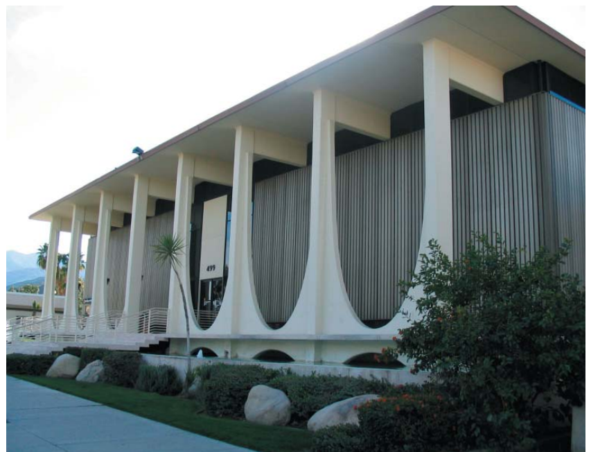
Top & Bottom: The eclectic collection of Spanish Colonial, Mediterranean, and Modern architectural styles in downtown Palm Springs is a valuable asset. New buildings should strive for excellence in architectural design while preserving or adding to the eclectic nature of downtown.
