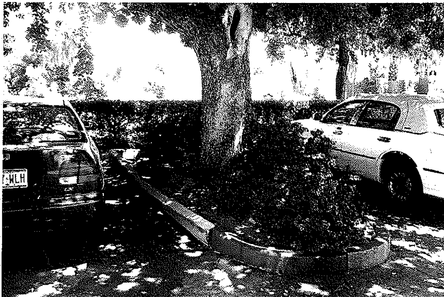
Curb Uplift and Water Run-Off Ponding
