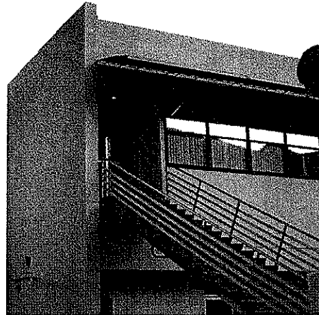
PORTION OF THE WEST FAÇADE SHOWING THE SHADE AWNING THAT WAS TORN OFF THE BUILDING IN HIGH WINDS EARLIER THIS YEAR; THIS AWNING WILL BE REPLICATED AND REPLACED.
