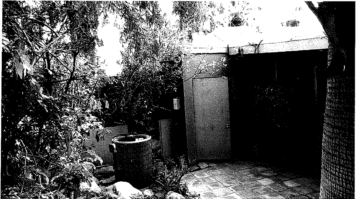
NORTH ELEVATION - VIEW LOOKING TOWARD EAST
