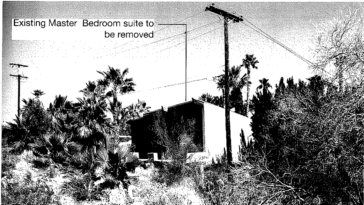
EXIST. MASTER BEDROOM SUITE - SOUTHWEST CORNER
