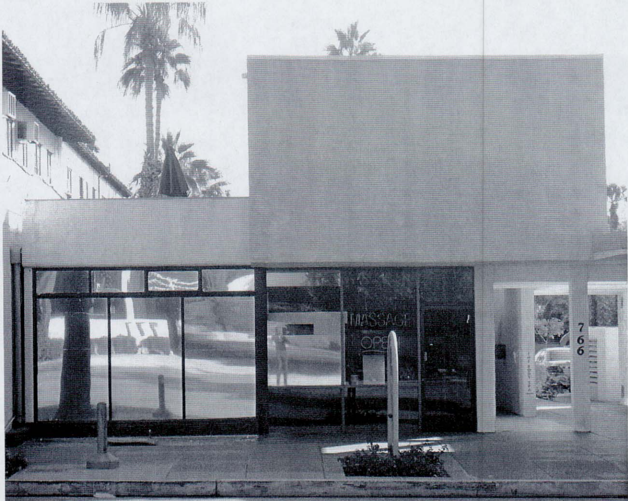
Figure 7 In this 2008 photograph, insensitive alterations conceal the largely intact primary facade of the building. A sensitive removal of the inappropriate alterations and restoration of the building's original character-defining spatial concepts could restore the building's original appearance and reconfirm its importance as Palm Springs first International Style building.
