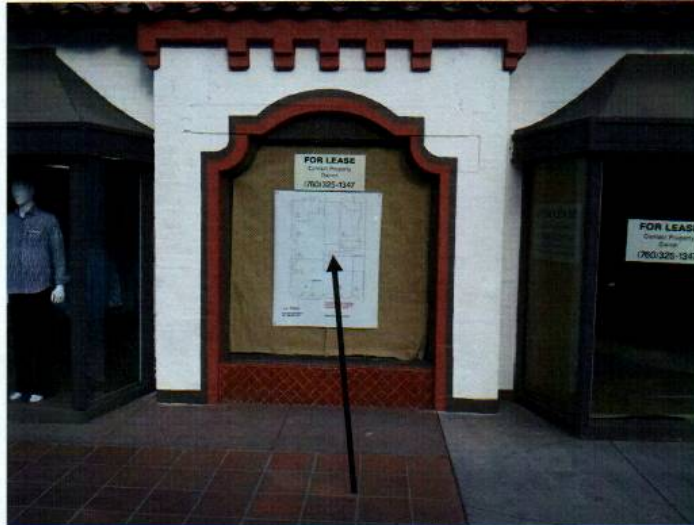
Location of Door "B"
