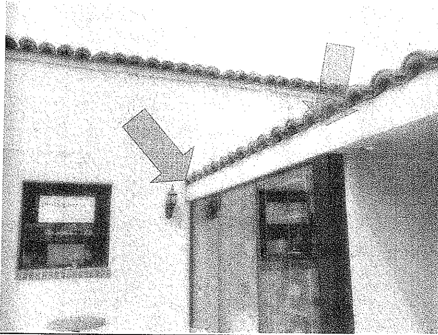
PHOTO 7 – Courtyard south window leaked due to reverse lap installation of the stucco band. Install a new drip flashing over the roof edge.
