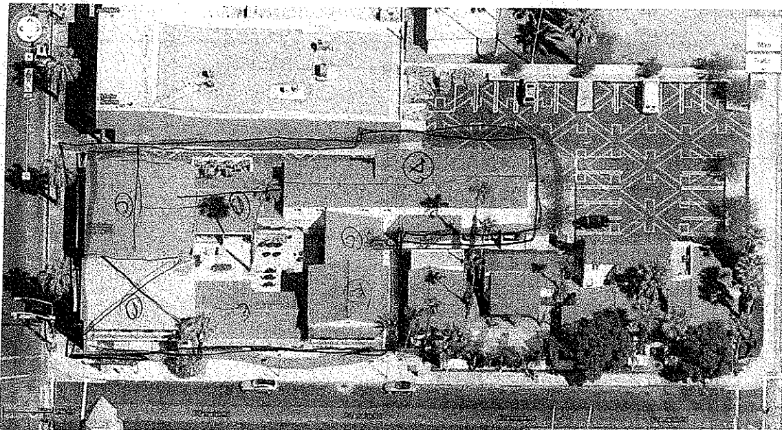
AERIAL VIEW OF SITE
