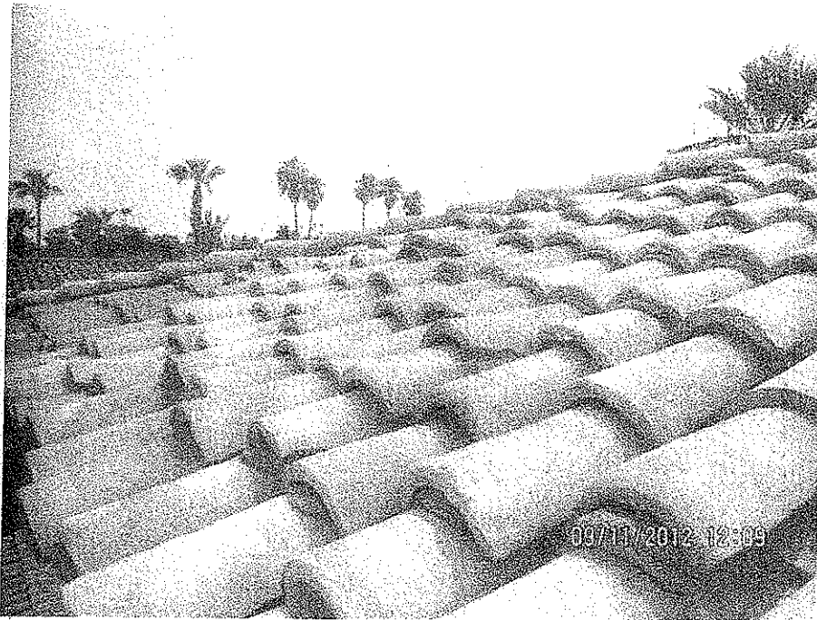
PHOTO 2 - Roof Suite B. historical designation of existing roof tiles by the City of Palm Springs.
