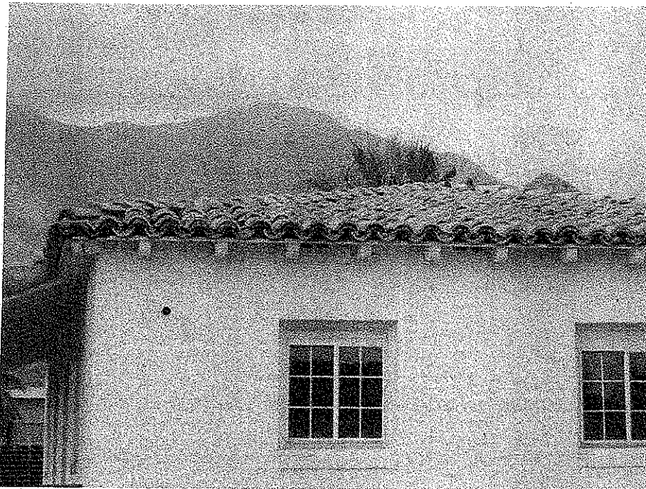
PHOTO 1 - South exterior elevation Suite B
