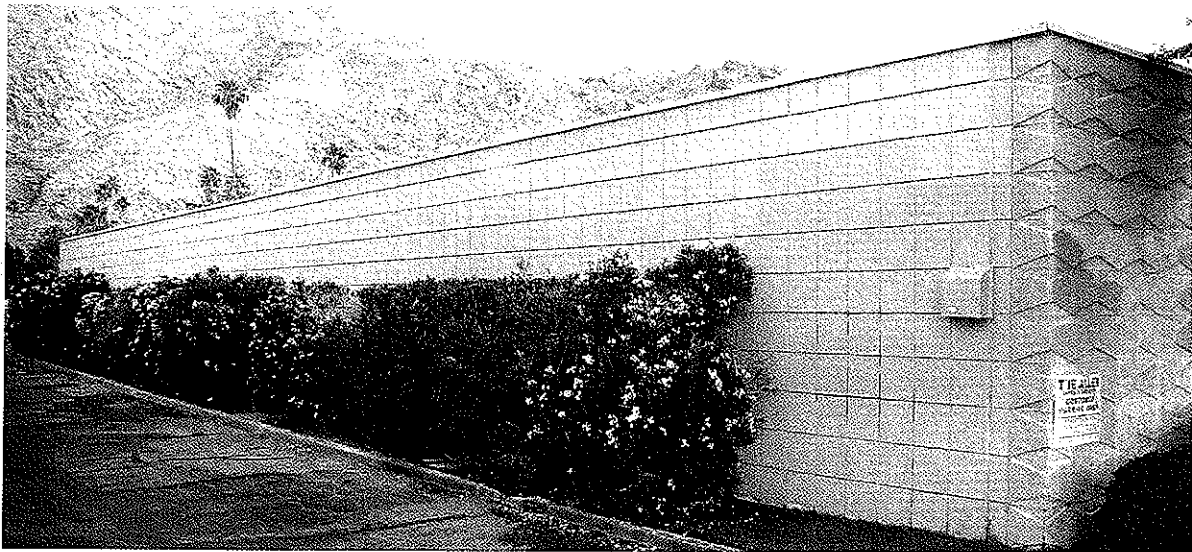
Figure 4: South elevation (southeast corner) (2012)
