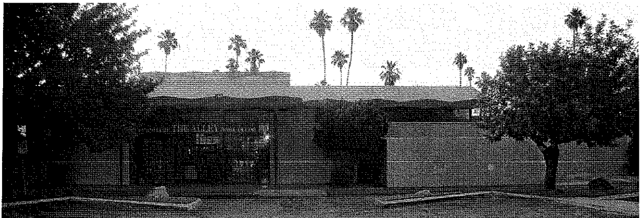
Figure 6: West elevation (southwest corner) (2012)
