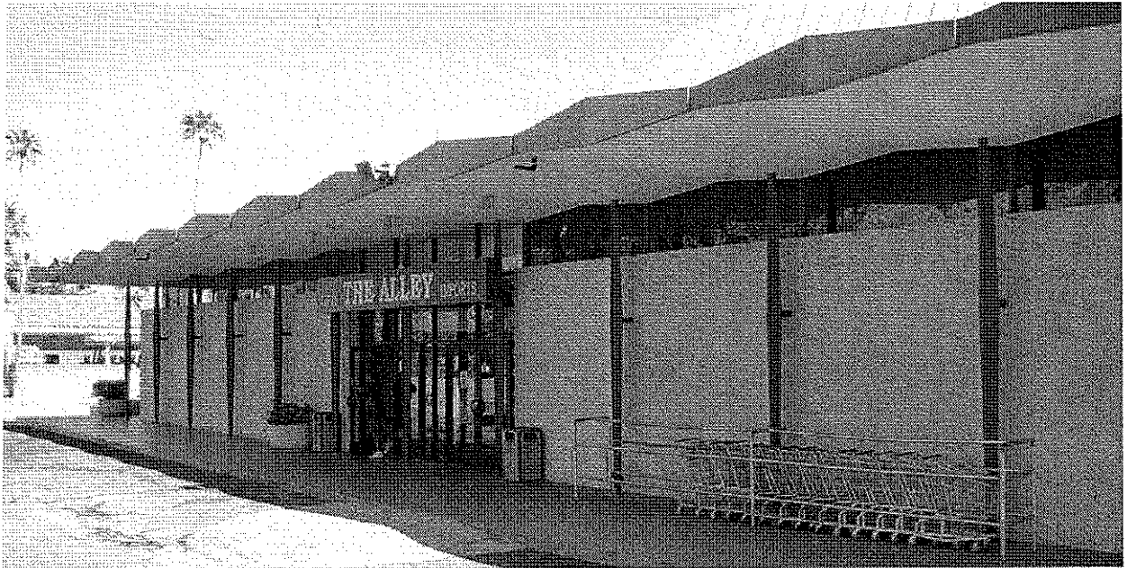
Figure 5: West elevation (northwest corner) (2012)
