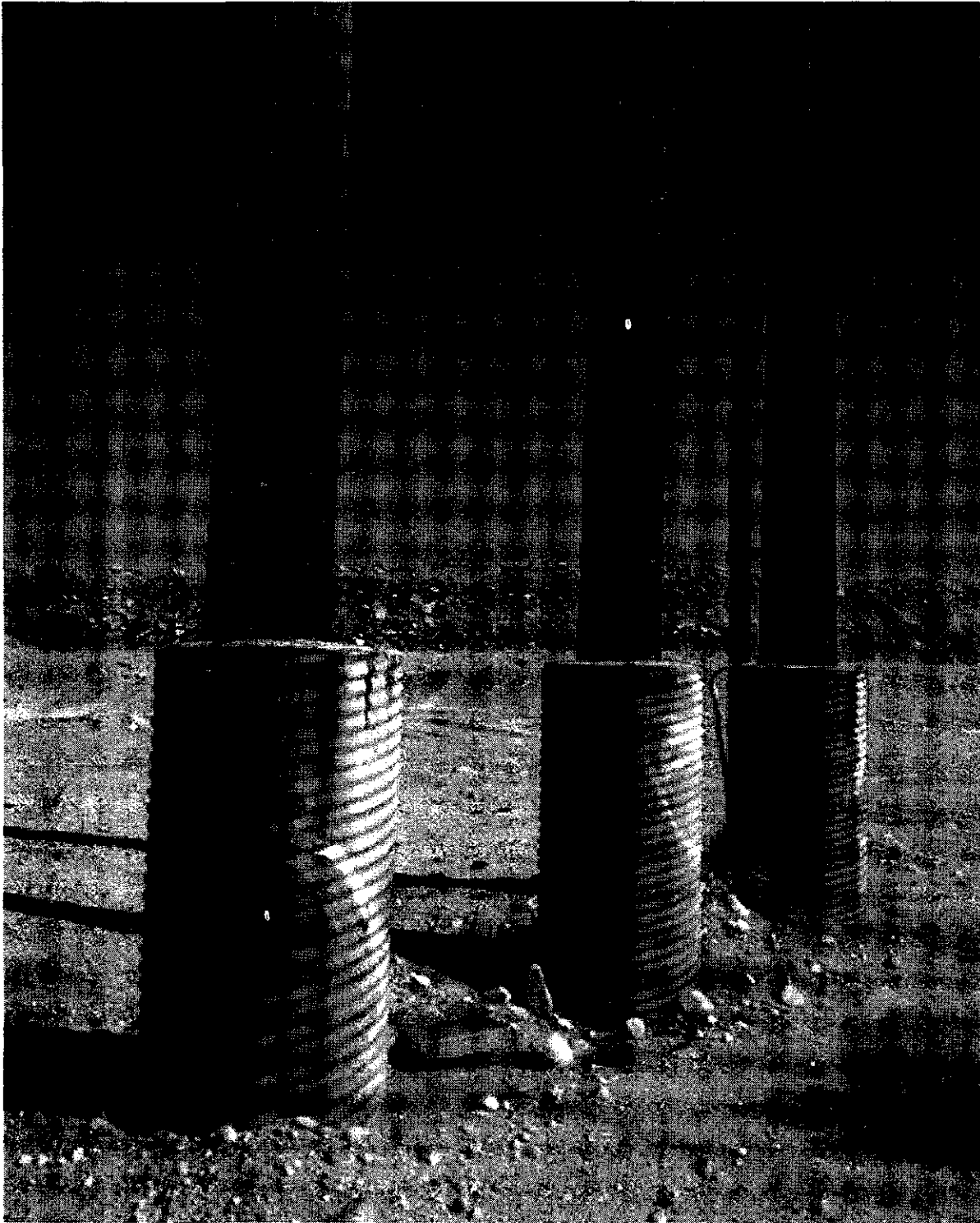
Base of large Structures – concrete
