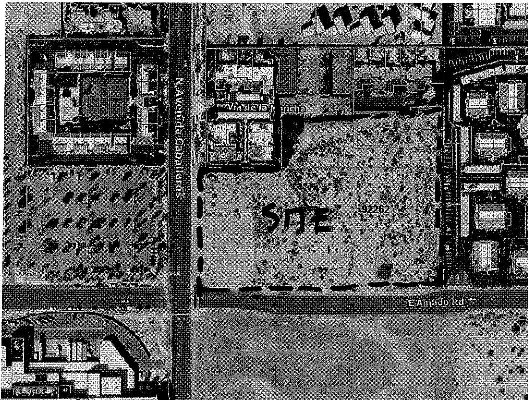
Aeria photo of project site
