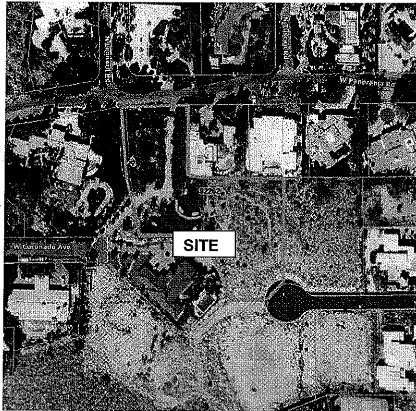
AERIAL PHOTO OF 801 PANORAMA ROAD
