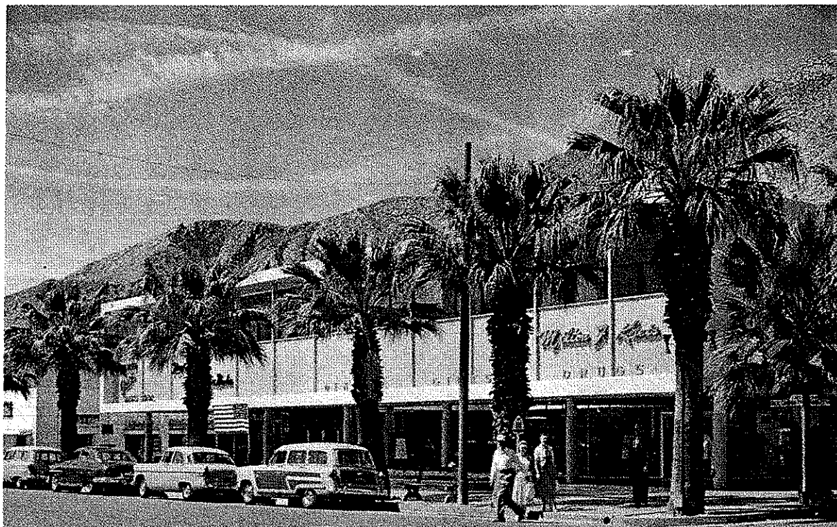
IMAGE c. 1954 – THE OASIS COMMERCIAL BUILDING
