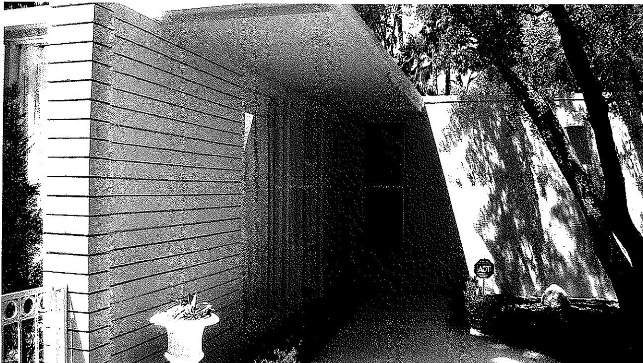
Figure 11. Roof eave detail designed for sun control
