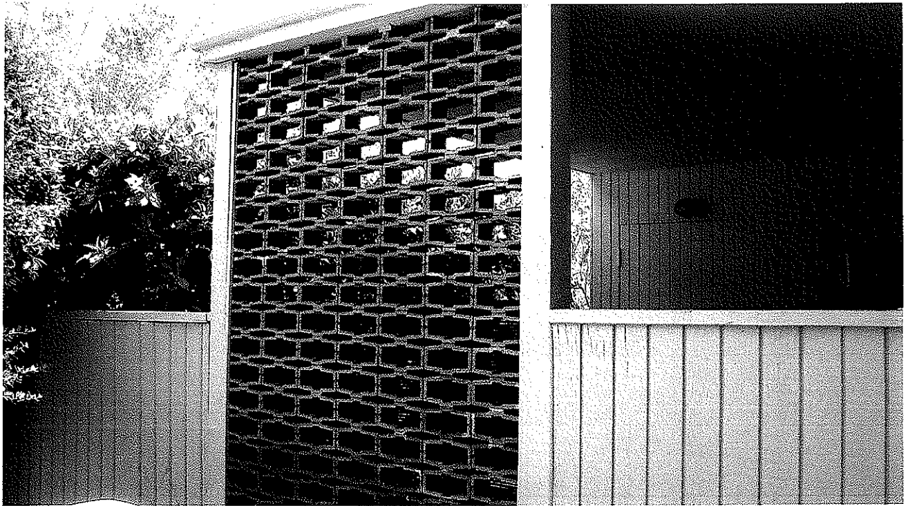
Figure 5. Occasionally, and possibly in conjunction with Bachelor units only, Cody's concrete block design is laid horizontally creating an interesting variation of the pattern.
