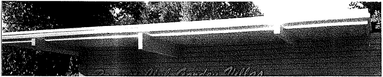
THIS MOTIF OF "SHORT-DEEP-SHORT" CANTILEVERED BEAMS OCCURS IN NUMEROUS LOCATIONS THROUGHOUT THE DISTRICT
