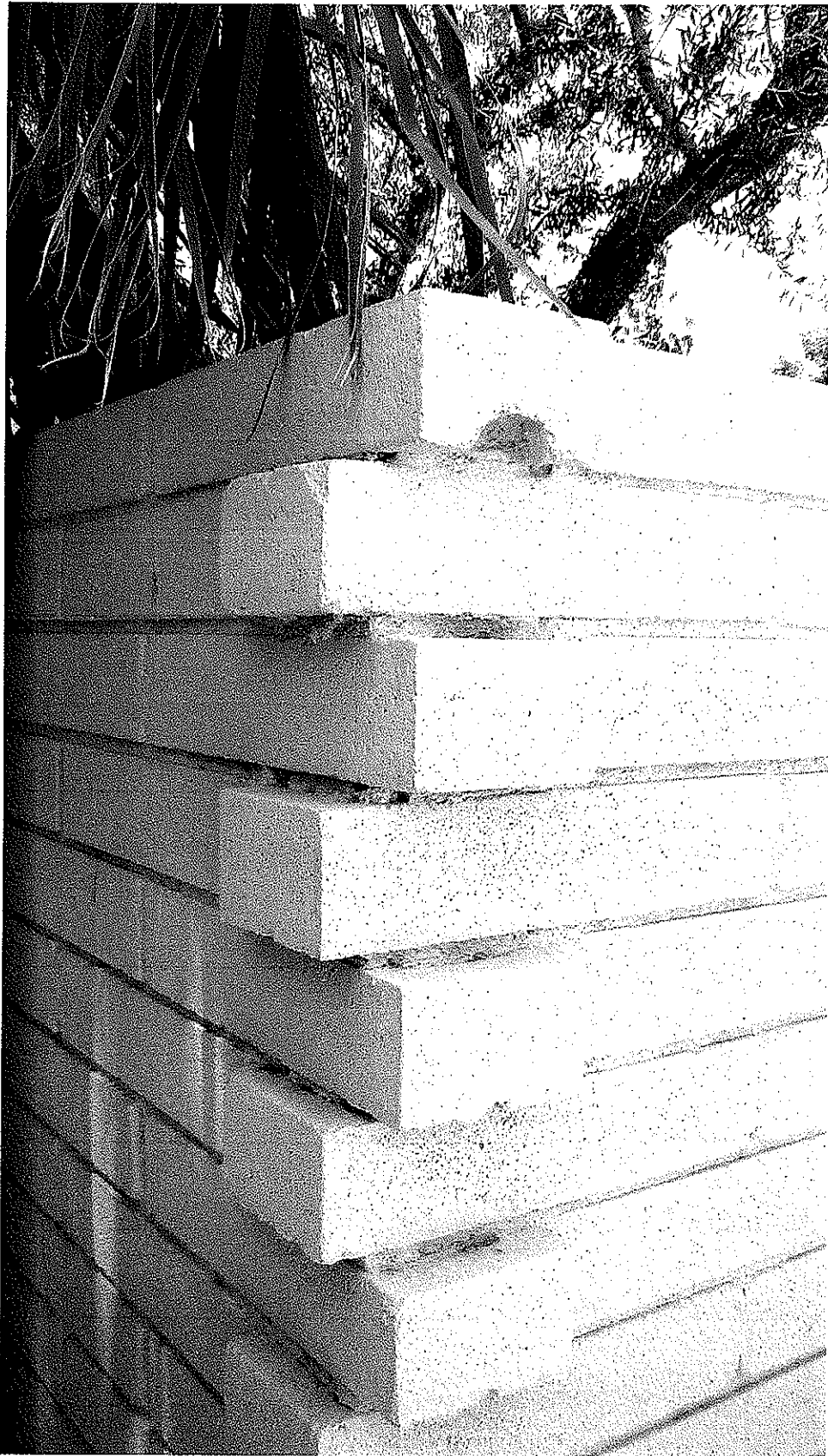
Figure 9. Cody's idiosyncratic use of concrete block in the RCCW complex includes some clever corner details.
