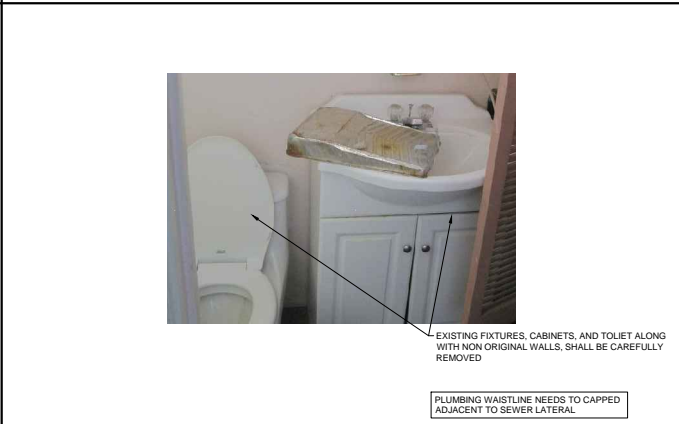
18 CARPORT CONVERSION BATHROOM INTERIOR
