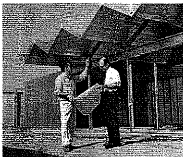
EARLY PHOTOS SHOWING CONSTRUCTION OF THE FOLDED PLATE ROOFED STEEL HOME.
