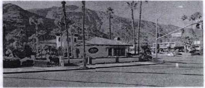
EXISTING VIEW NW CORNER OF S PALM CANYON DRIVE & MORONGO ROAD
