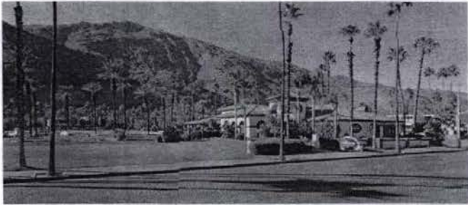
EXISTING VIEW NW ALONG S PALM CANYON DRIVE
