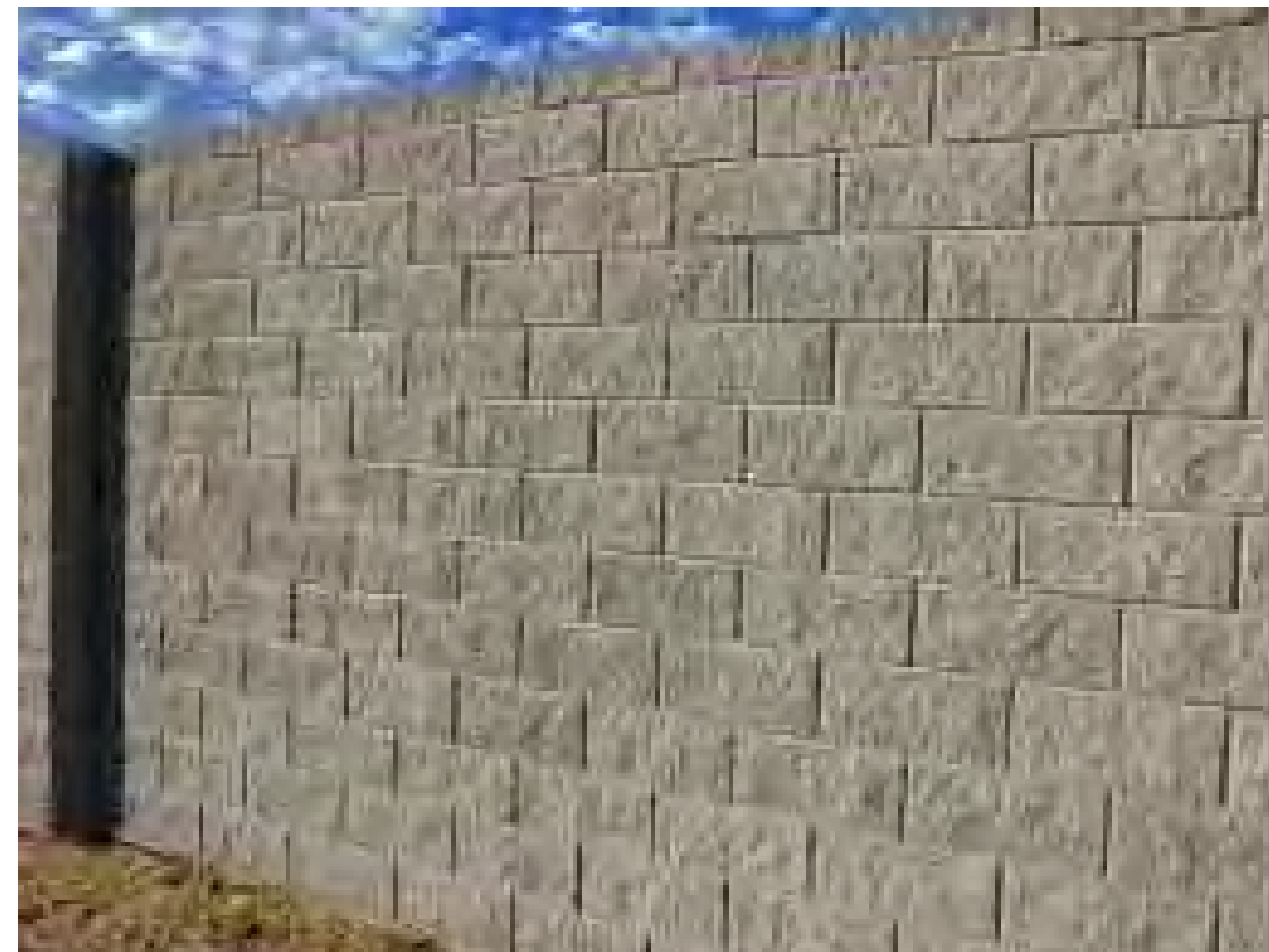
SPLIT-FACE CMU WALL
