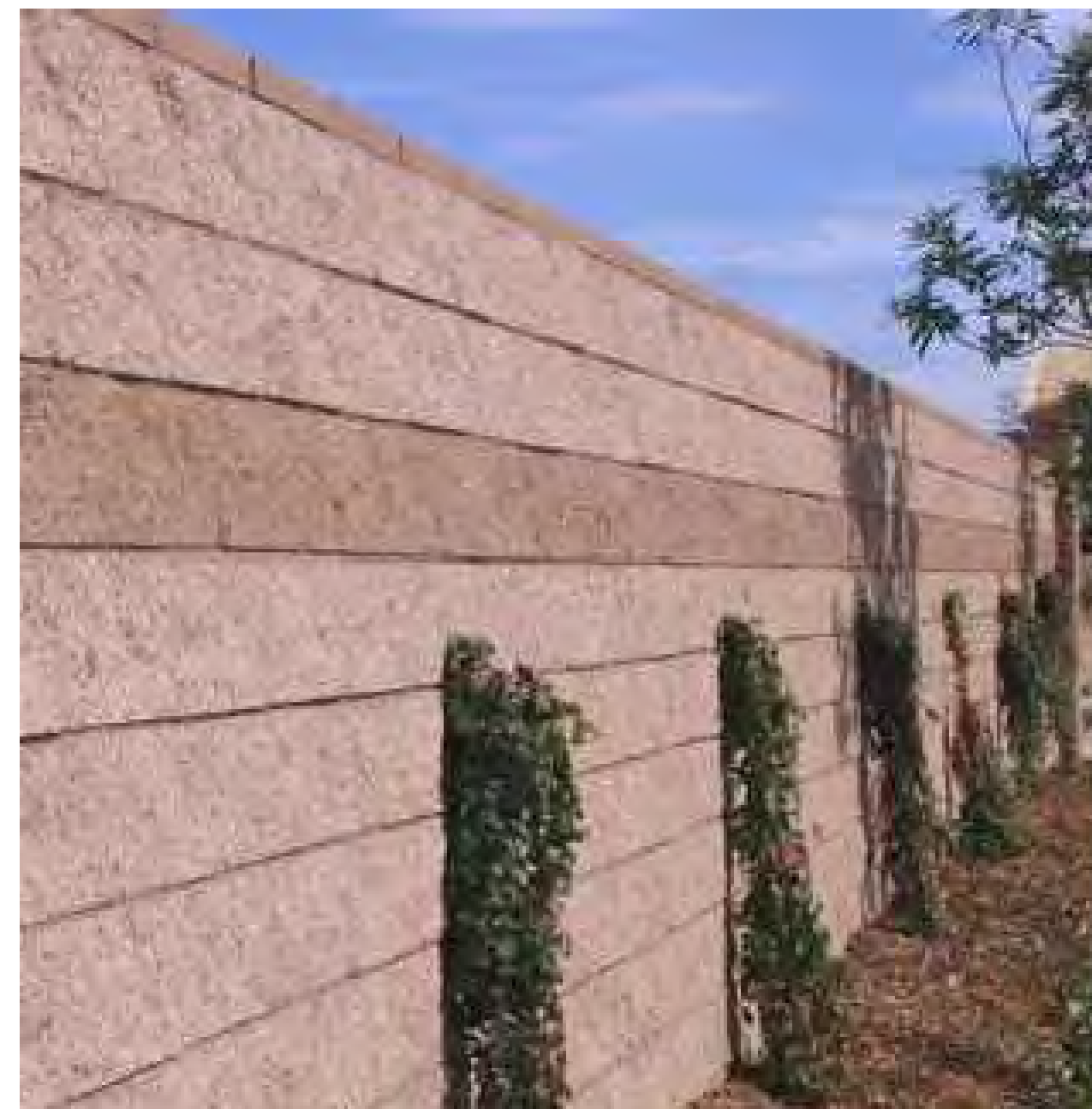
SPLIT-FACE CMU WALL WITH PLANTING
