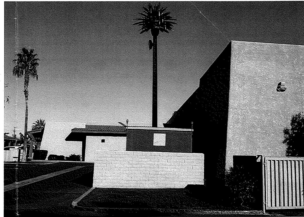
PROPOSED INSTALLATION OF 60' MONOPALM WITH ANTENNA ARRAY AND ADDITION TO EXISTING EQUIPMENT COMPOUND (ADDITION TO COMPOUND NOT VISIBLE FROM THIS VIEW).
