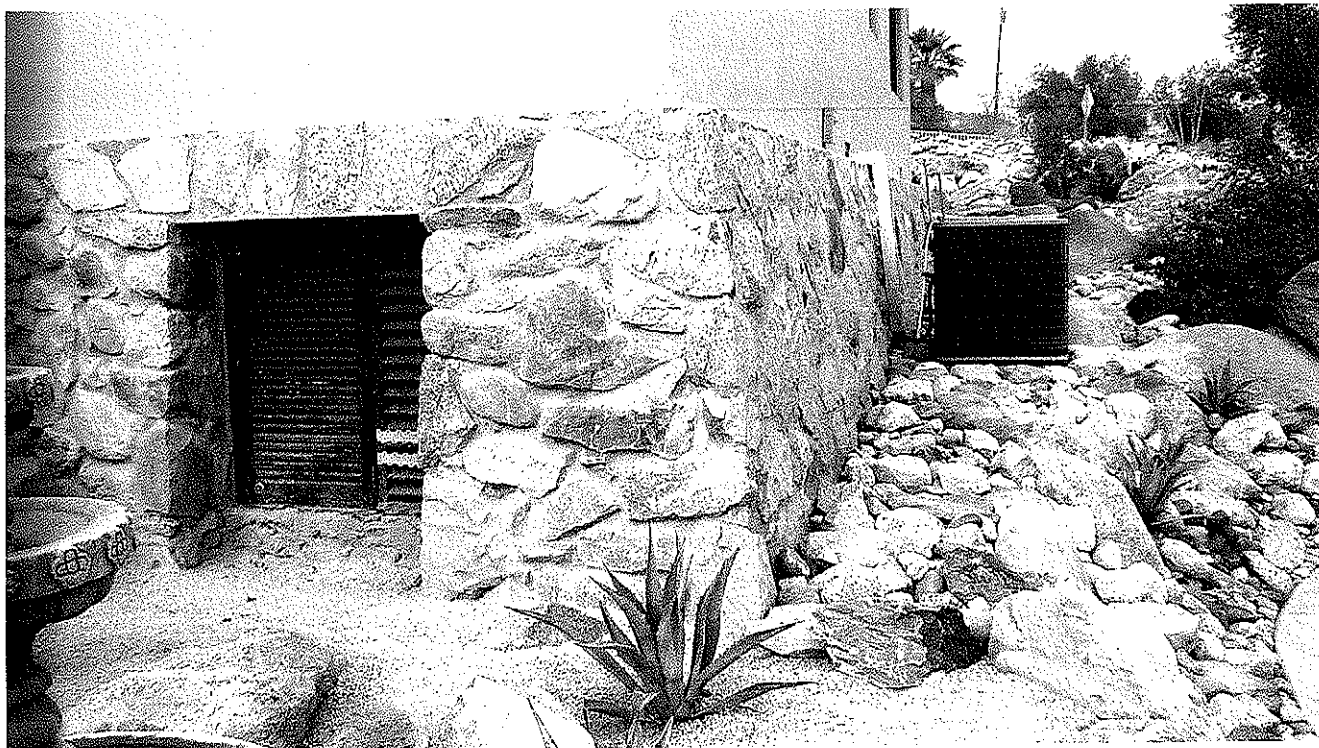
Stem Walls Form a 7-foot high Underfloor Area Entered Through an Access Door
