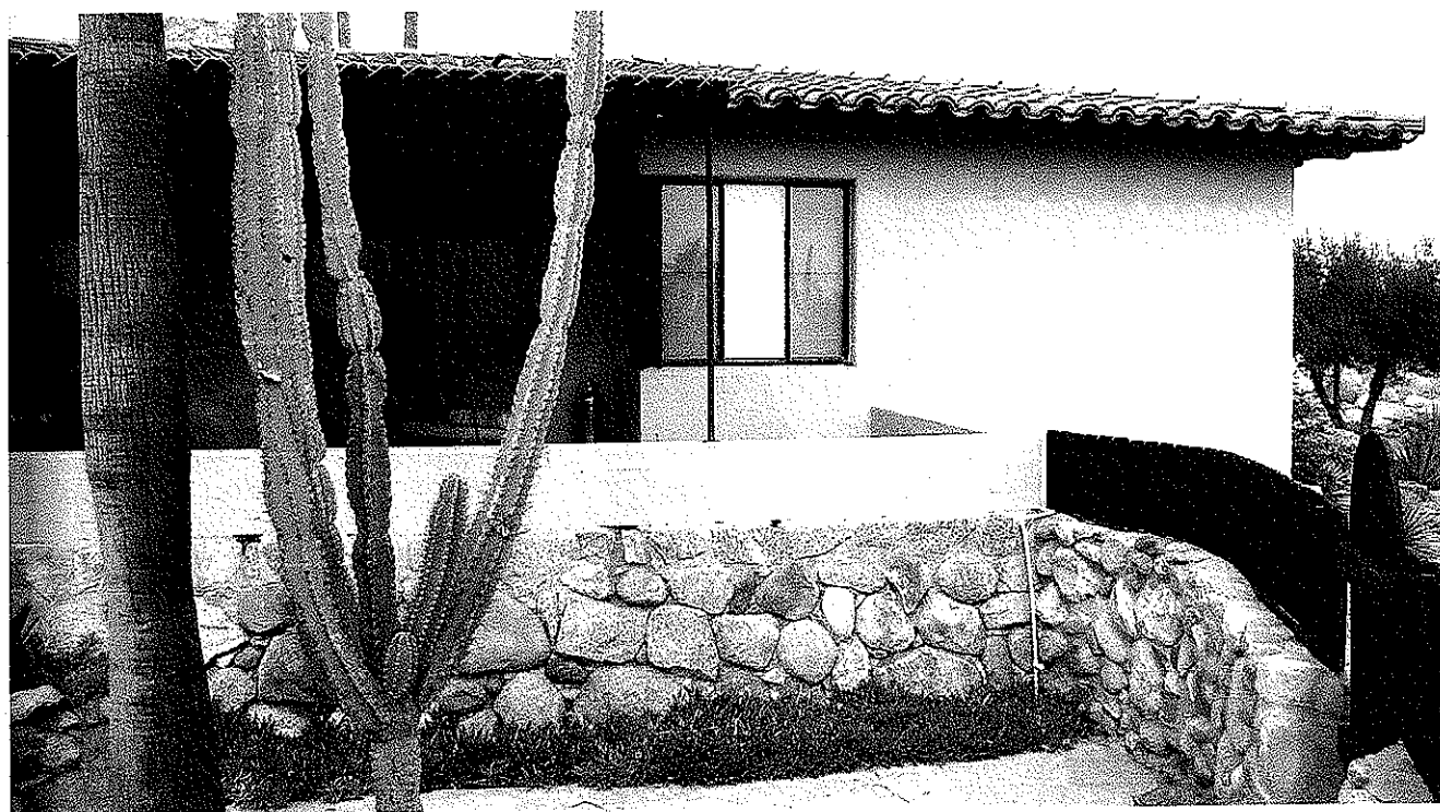
Native Stone Walls Topped with Concrete Block Enclosing Rear Patio Area
