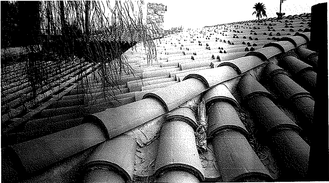
Terra Cotta Barrel Tile Hip Roof
