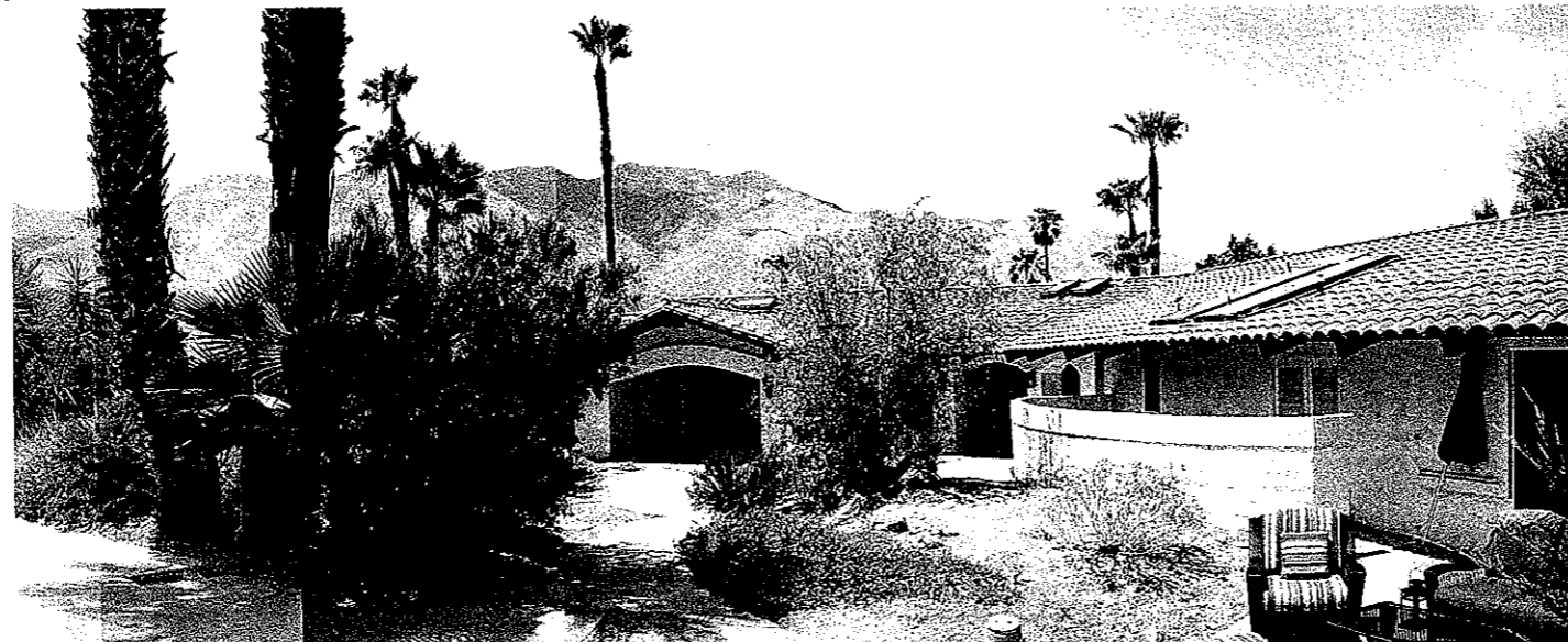
View to West showing existing entryway featuring shallow arches.
