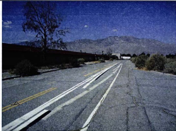
Photo No. 25 – West view of unused roadway north of self-storage buildings.
