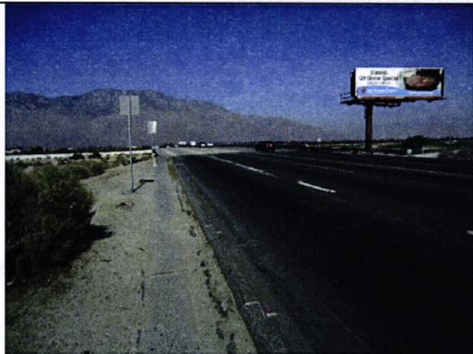
Photo No. 3 – West view of Ramon Road before bridge.
