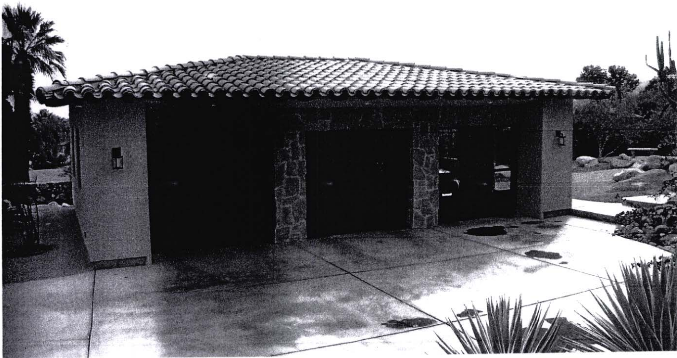
Non-Contributing Three-Bay Garage Building with Barrel Tile Hip-Roof Built in 2010. The New Garage Emulates the Main Residence in Design and Materials.
