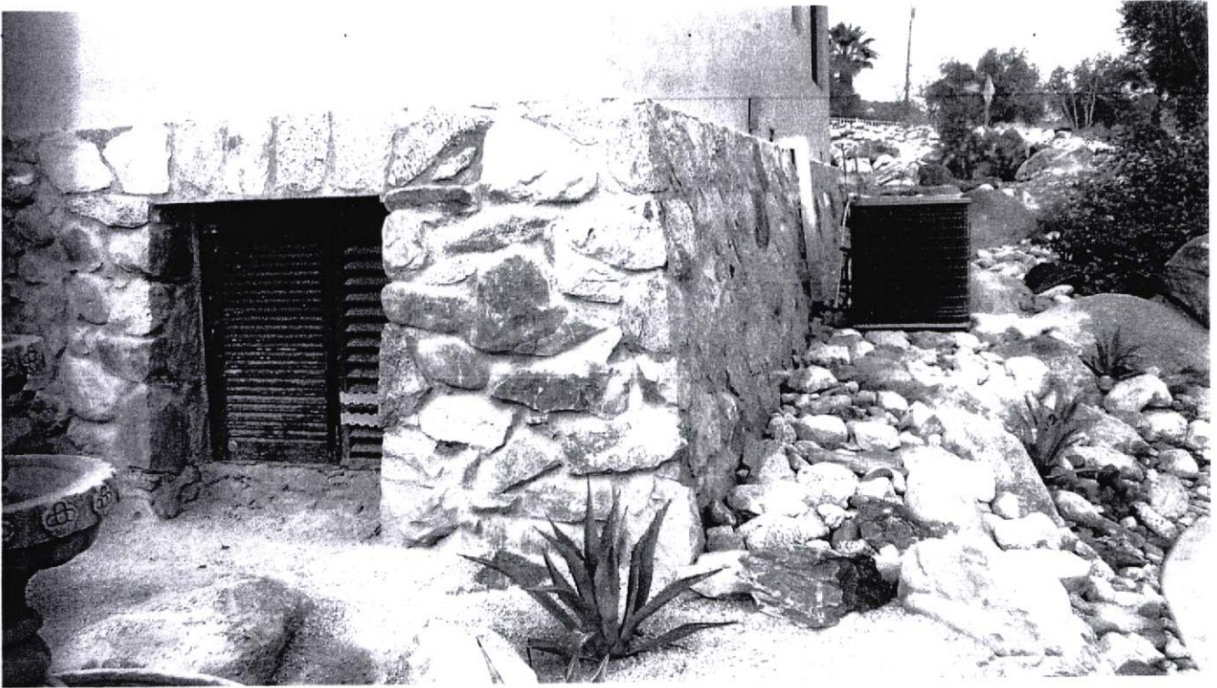
Stem Walls Form a 7-foot high Underfloor Area Entered Through an Access Door
