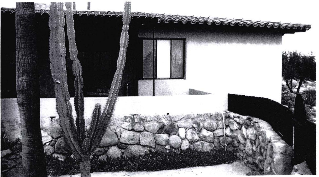
Native Stone Walls Topped with Concrete Block Enclosing Rear Patio Area
