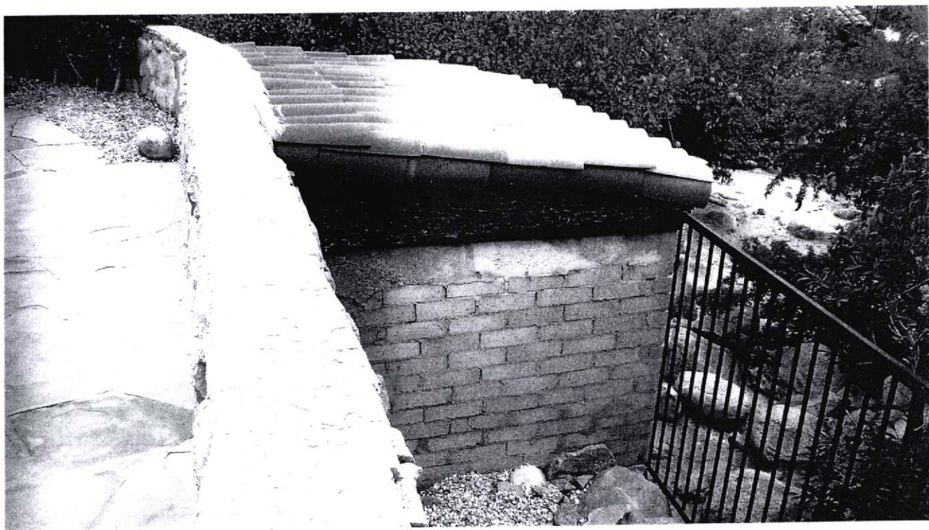
Non-Contributing Pool Equipment Building with Barrel Tile Shed Roof
