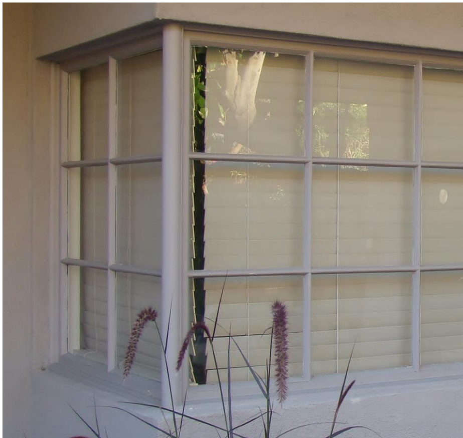
Metal casement windows meeting at a corner with metal pipe support
