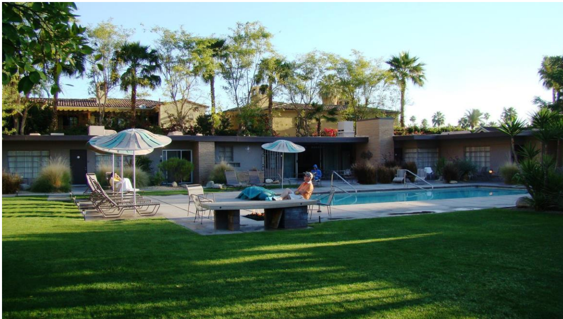
The south and east façades of the Town & Desert Apartments Courtyard
