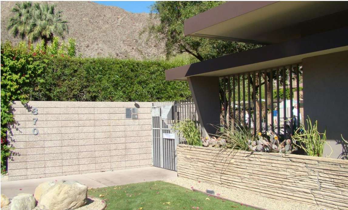
The south façade of the Town & Desert Apartments showing 2001 additions (block wall and steel gate structure) made to control access. Also shown is the mortared stacked sandstone wall, laid ledge-style, creating a planter structure and vertical wood brise-soleil . Note the artistic perpendicular intersection of the roof planes.
