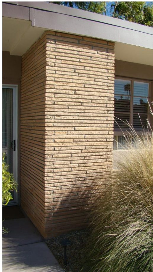
Stacked sandstone pier supporting the roofline plane
