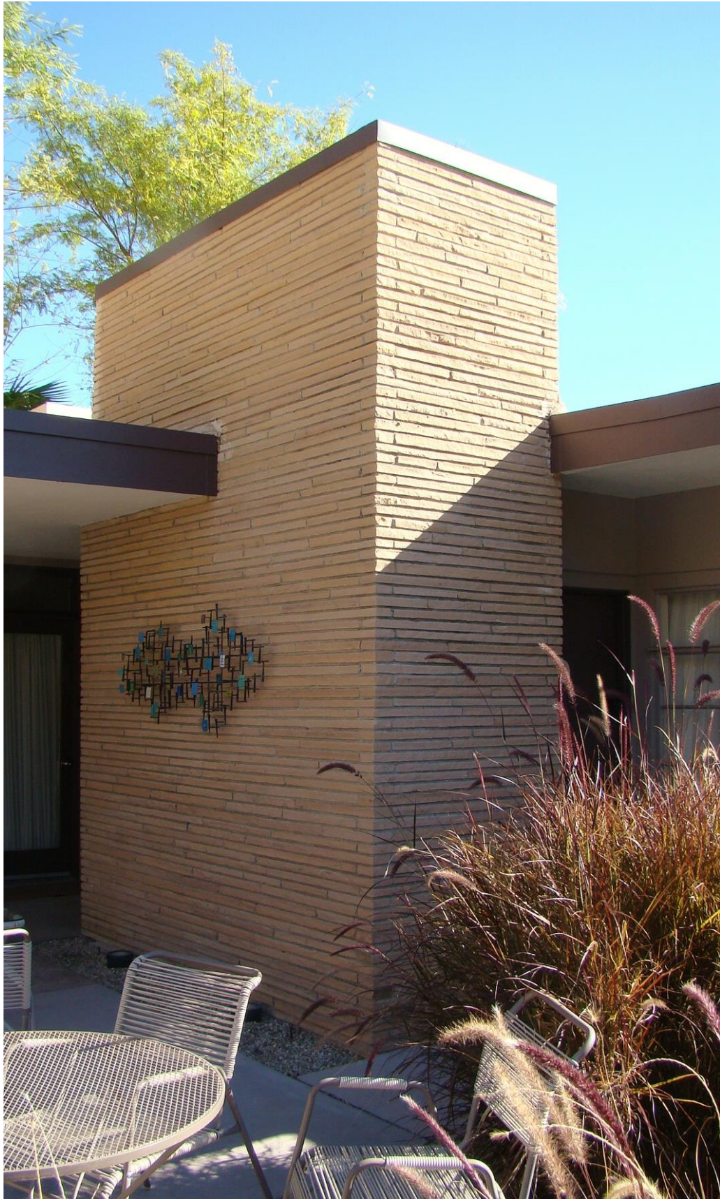
Stacked sandstone pier piercing the roofline
