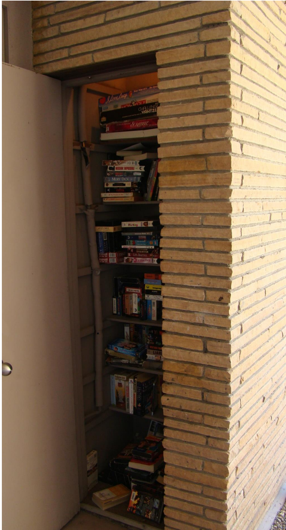
Stacked sandstone pier housing outdoor storage space
