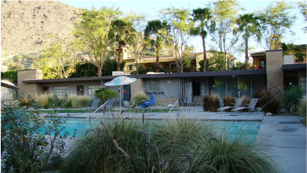
The south courtyard façade of the Town & Desert Apartments
