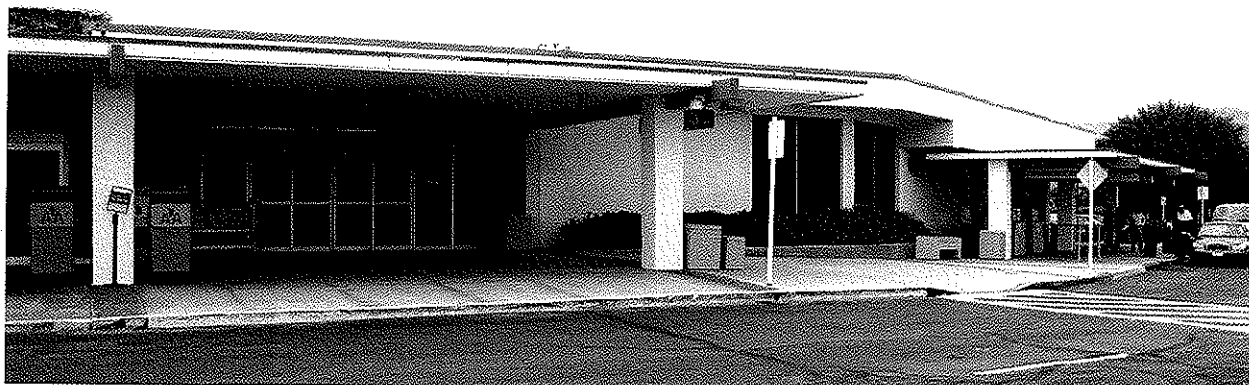
South end of Ticketing area
