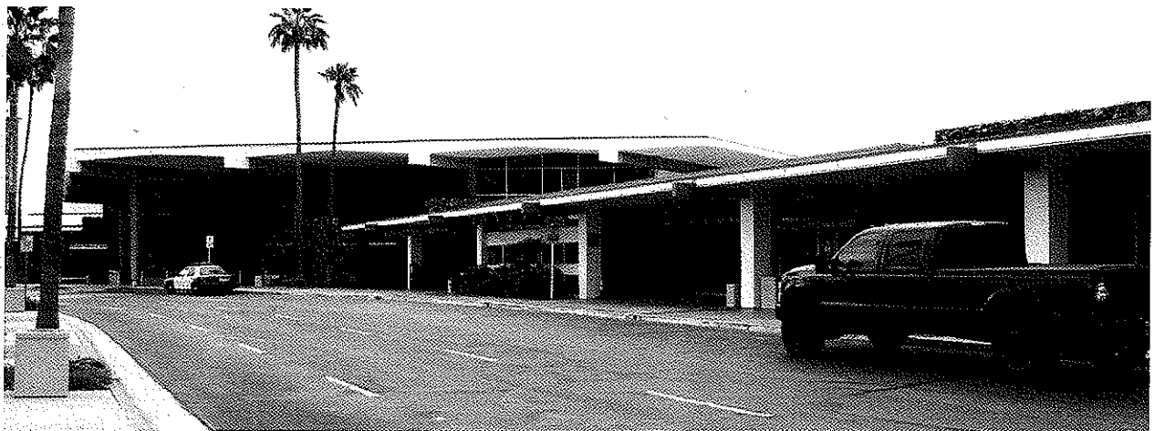
Main Entrance and Ticketing area
