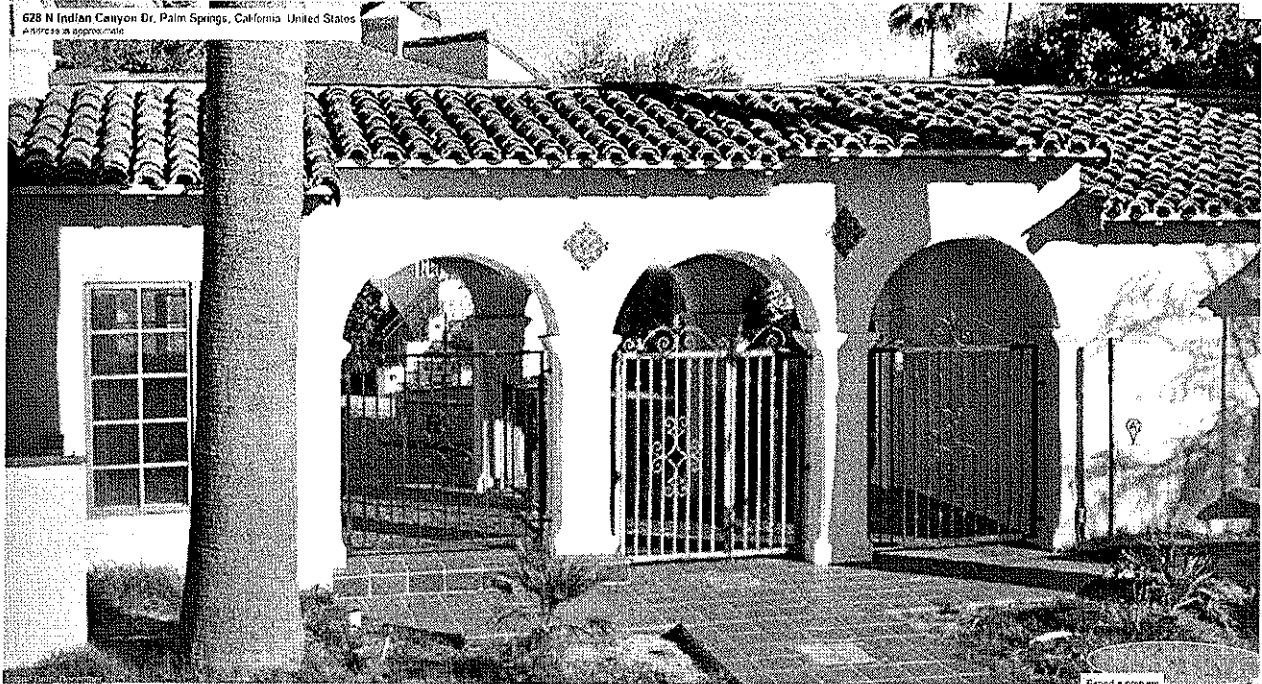
EXISTING ARCHED ARCADE PORCH ALONG INDIAN CANYON DRIVE
