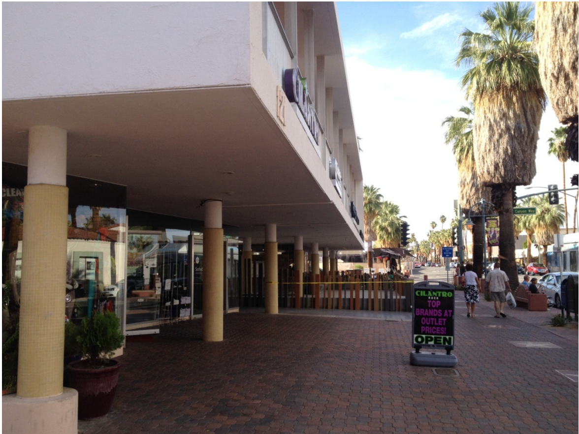
Southeast Corner Elevation
