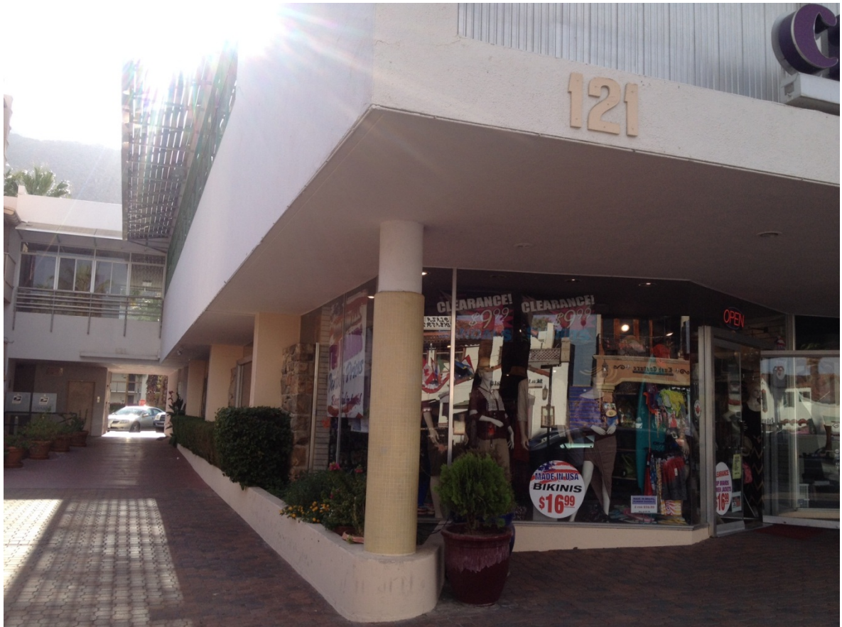
Southeast Corner Elevation
