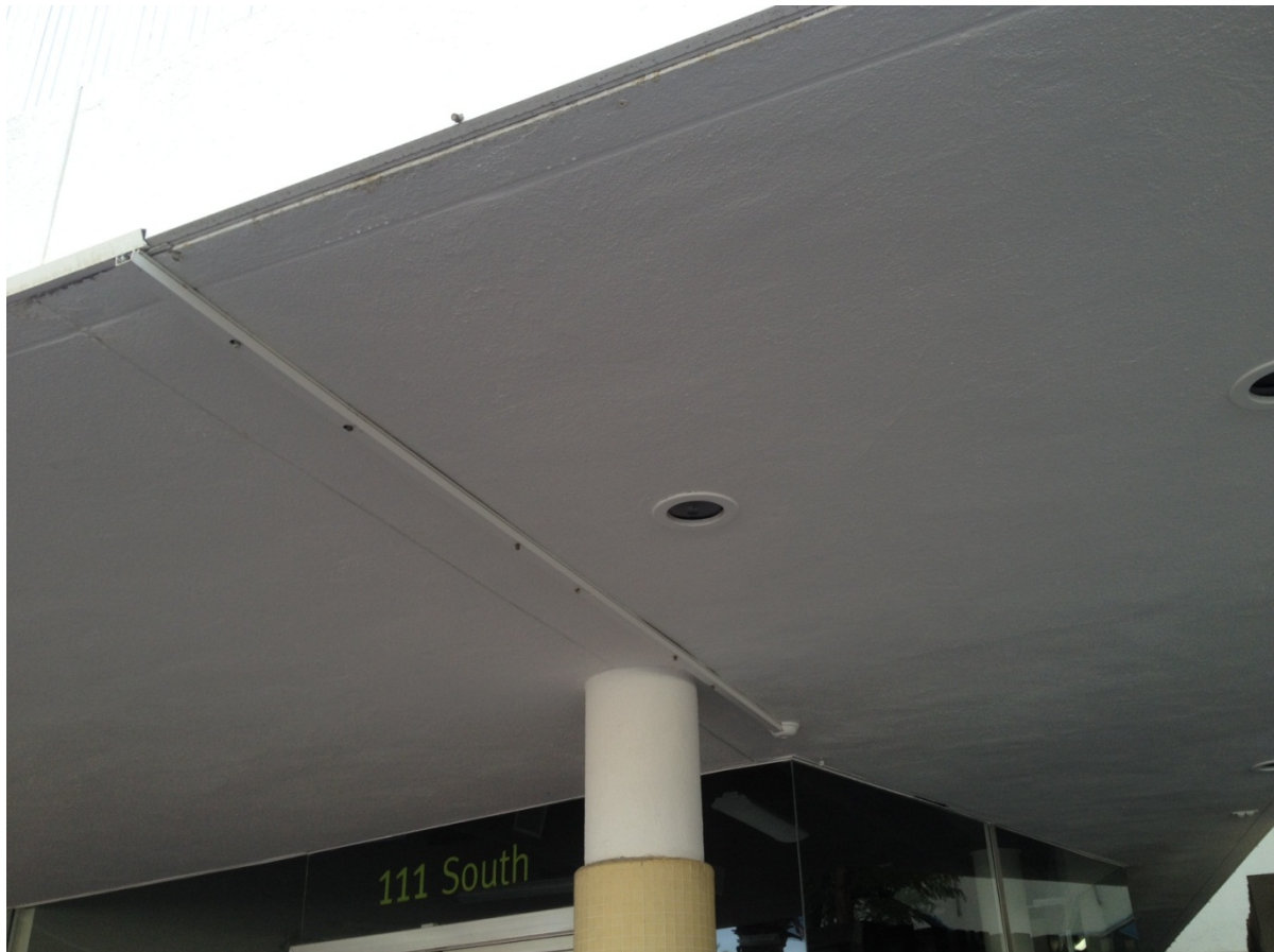
East Elevation Soffit
