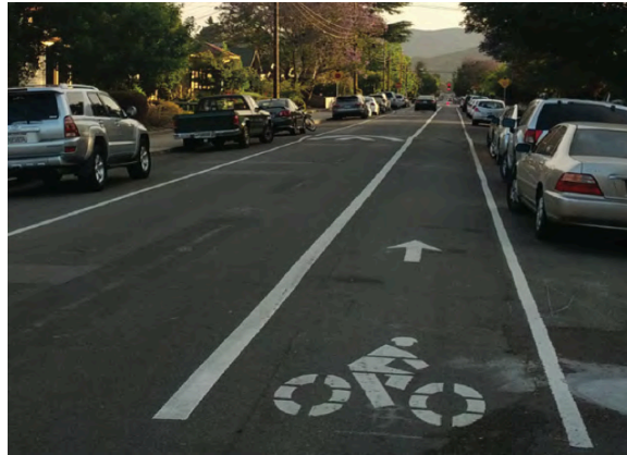
FIGURE 8 Bike lane striping and stencil.
