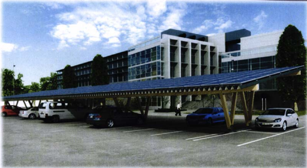
Parking Lot Non-traditional Fix Tilt Solar System
