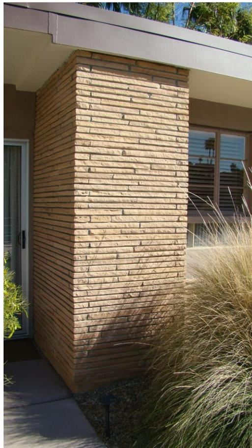
**Stacked sandstone pier supporting the roofline plane**
