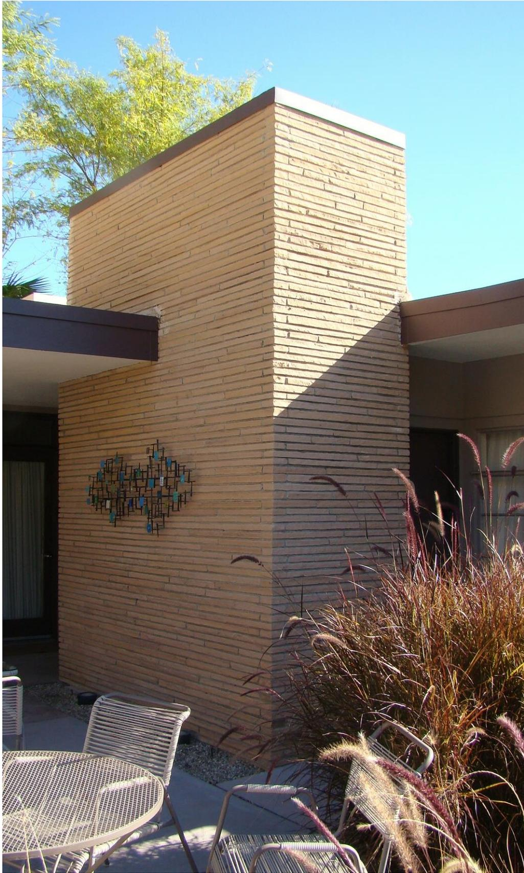
**Stacked sandstone pier piercing the roofline**
