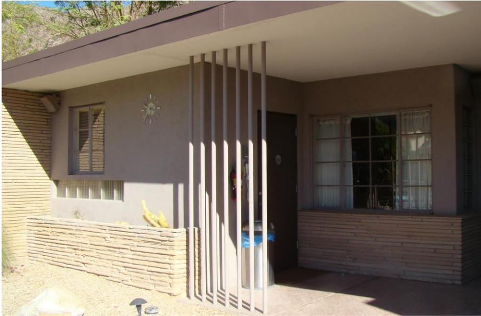
**Detail of mortared stacked sandstone planter (left), stacked sandstone pier (far left), stacked sandstone wainscoting (right), metal pipe supports (center), casement windows and glass block**
