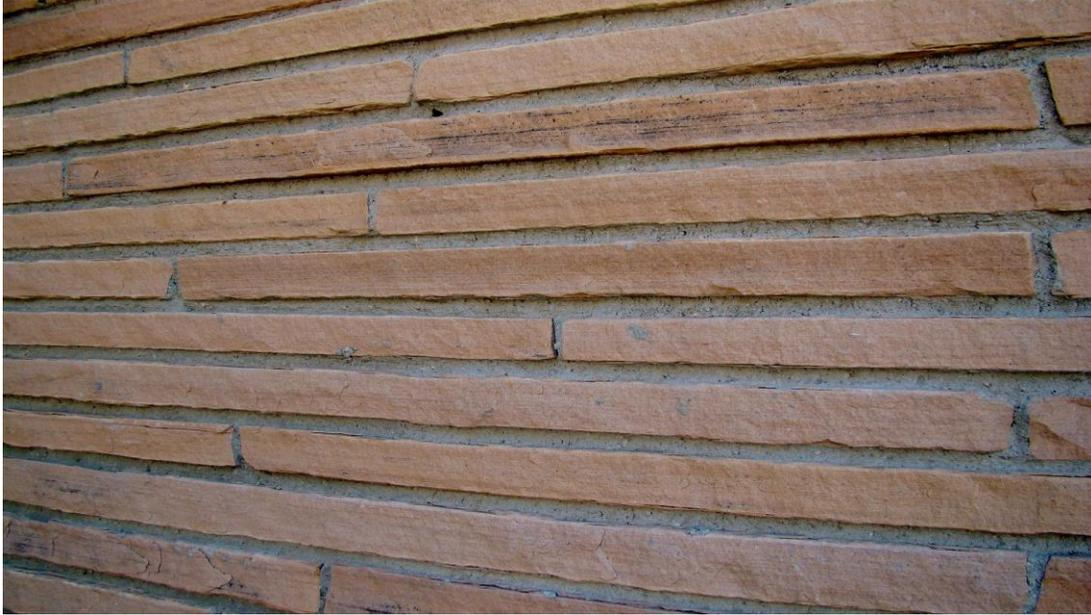
**Detail of mortared stacked sandstone laid ledge-style. The length of these sandstone slabs can vary from 4 inches to almost 36 inches**
