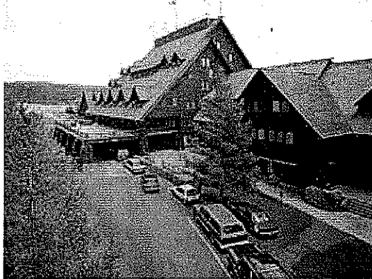
Old Faithful Inn, Yellowstone National Park, Wyoming brought the Rustic style to the West in 1903 in an original design, and a scale befitting its setting. Photo: Courtesy, Historic American Buildings Survey, NPS.
