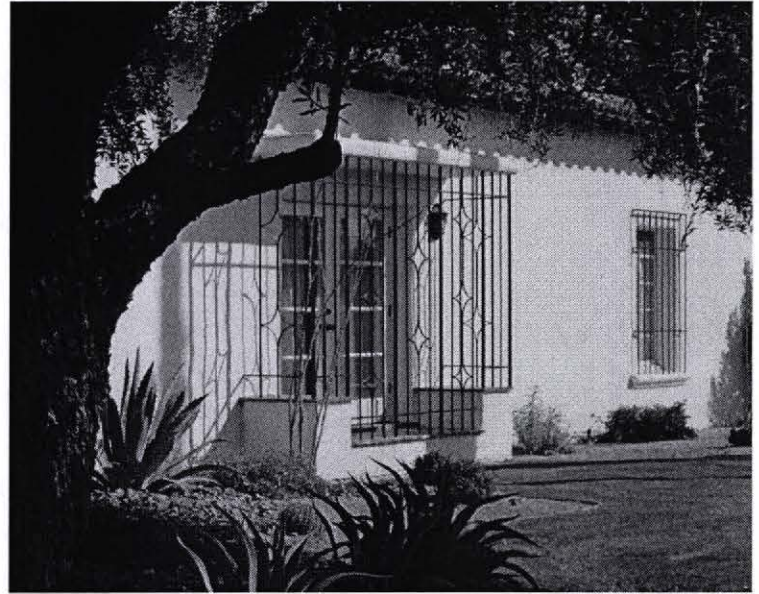
Balcony with wrought iron and extended stucco sill at window (main house).
