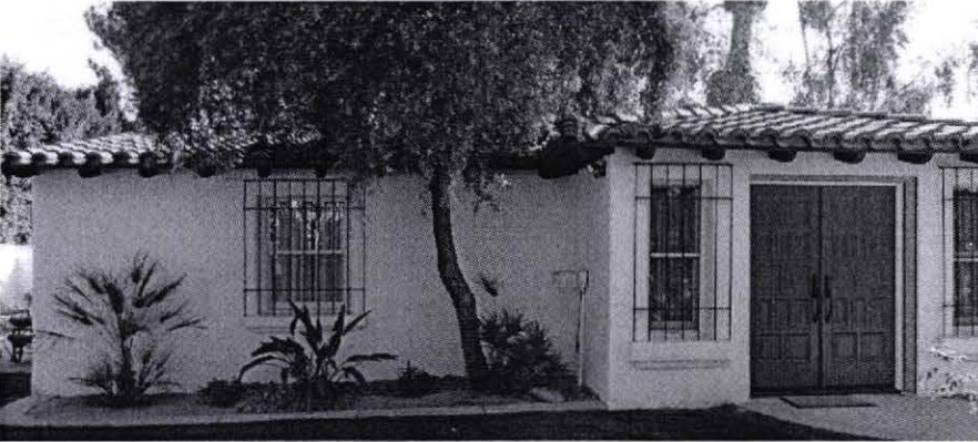
West façade of guest house (windows and doros not original)
