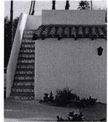
Stair at rear of main house to roof deck.
