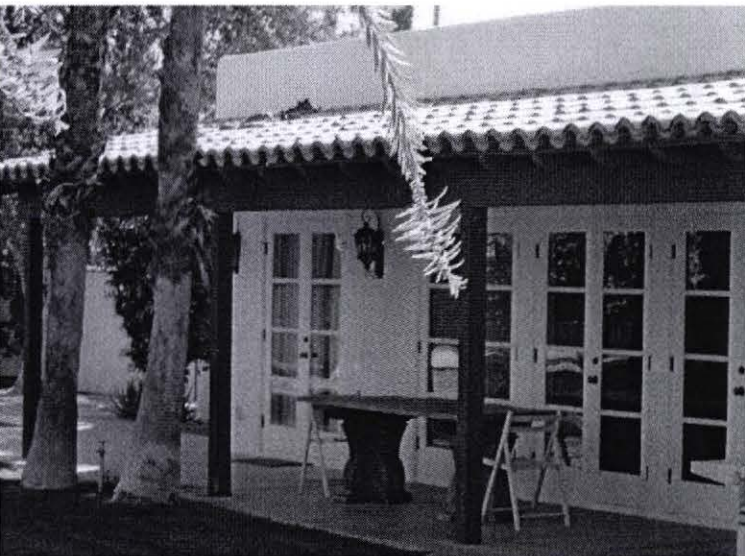
Rear covered patio of main house (roof and doors not original)
