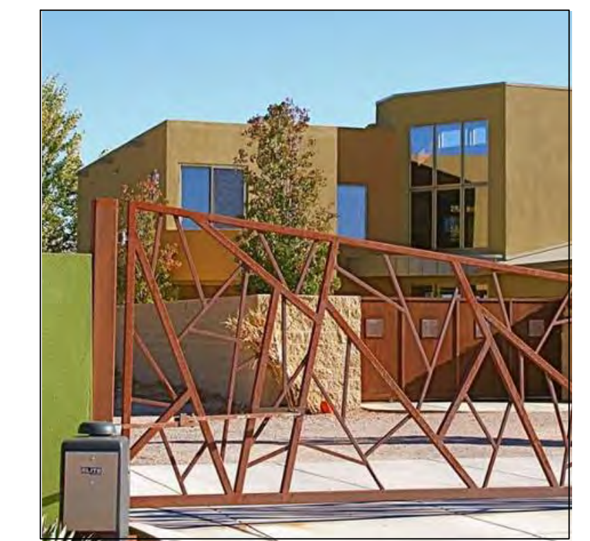
ENTRY GATE MANUFACTURER: UNKNOWN TYPE: TUBULAR STEEL COLOR: SW 2849 WESTCHESTER GRAY (INNER RAILS) COLOR: SW 2850 CHELSEA GRAY (OUTER RAILS)
