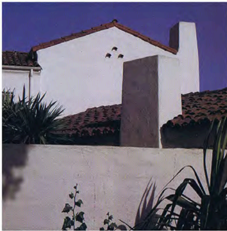
2 - STUCCO - HAND APPLIED STEEL TROWELED SMOOTH FINISH - MERLEX STUCCO SANTA BARBARA FINISH COLOR COAT STUCCO IN EL DORADO WHITE
