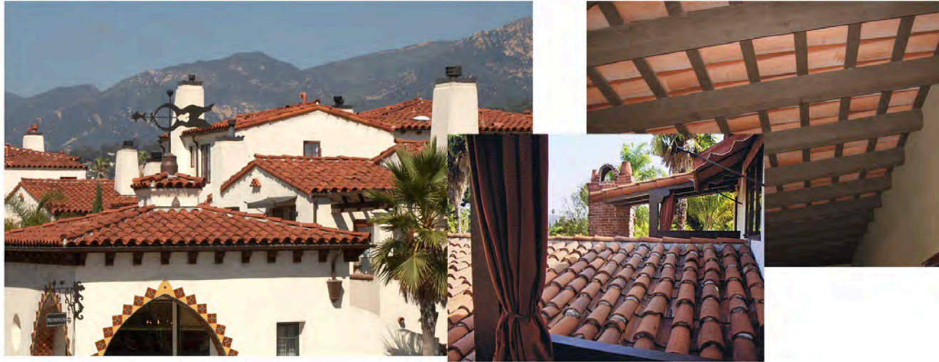
2 - STUCCO - HAND APPLIED STEEL TROWELED SMOOTH FINISH - MERLEX STUCCO SANTA BARBARA FINISH COLOR COAT STUCCO IN EL DORADO WHITE
