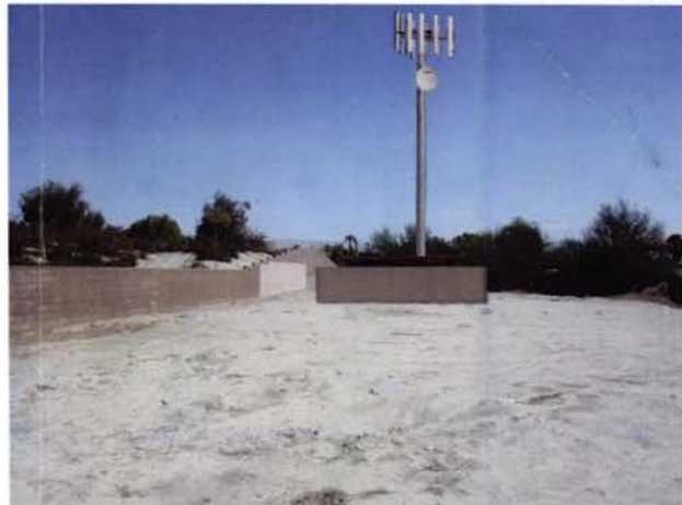
PROPOSED INSTALLATION OF 60' MONOPOLE WITH ANTENNA ARRAY AND RRU'S, INCLUDING EQUIPMENT COMPOUND WITH SHELTER, GENERATOR, AND 8' BRICK WALL.
