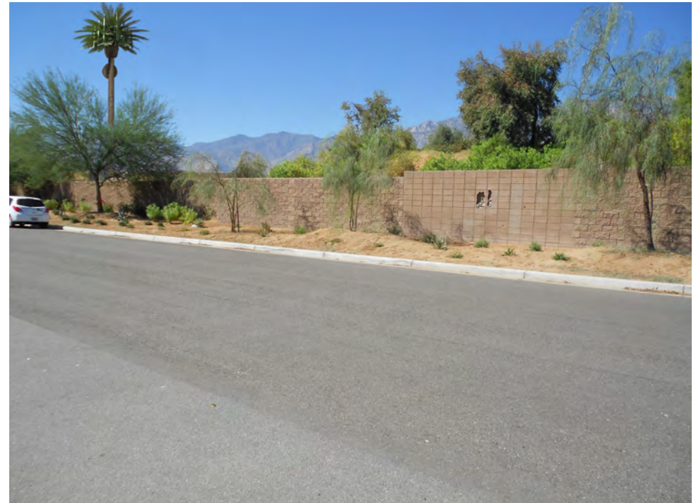
PROPOSED INSTALLATION OF 60' MONOPALM WITH ANTENNA ARRAY AND RRU'S, INCLUDING EQUIPMENT COMPOUND WITH SHELTER, GENERATOR, AND 8' BRICK WALL.
