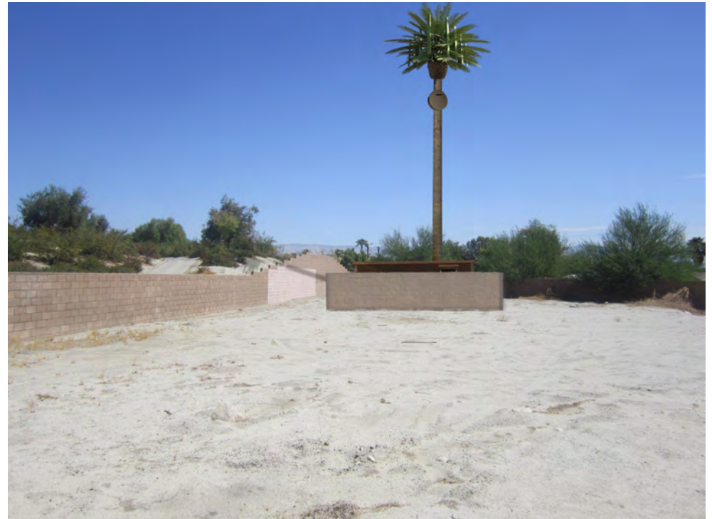
PROPOSED INSTALLATION OF 60' MONOPALM WITH ANTENNA ARRAY AND RRU'S, INCLUDING EQUIPMENT COMPOUND WITH SHELTER, GENERATOR, AND 8' BRICK WALL.
