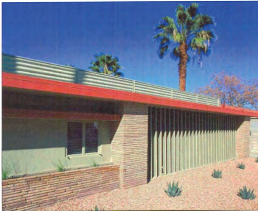
Village Manor exterior after restoration (Courtesy Orbit In Hotel)
