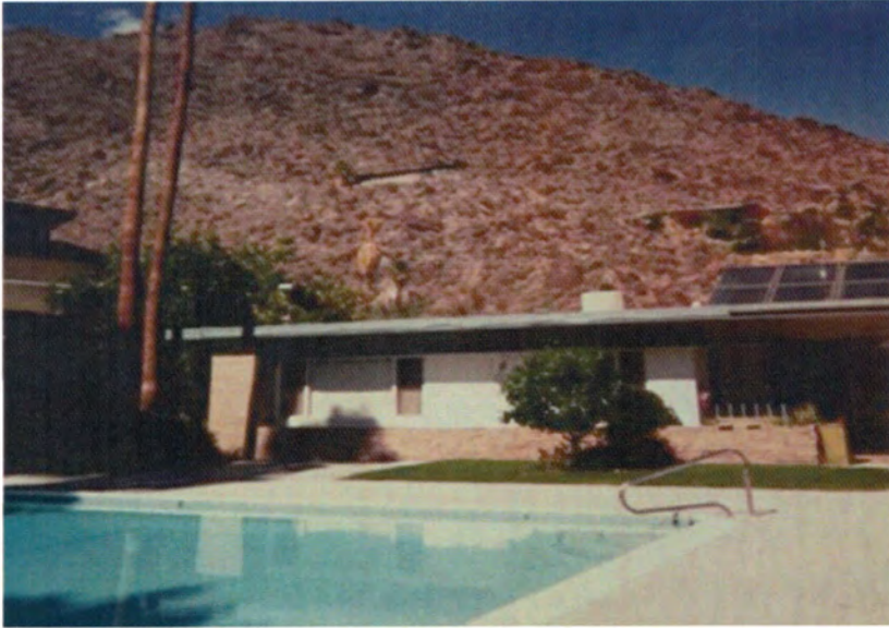
Photo by Christy Eugenis South-facing courtyard façade pre-restoration
