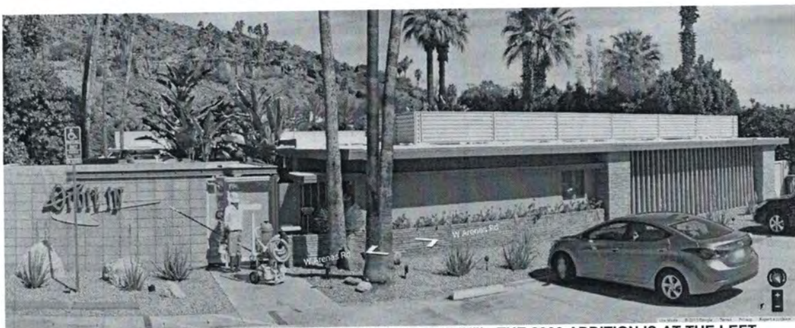
STREET ELEVATION OF VILLAGE MANOR (A.I.A. "ORBIT IN"). THE 2000 ADDITION IS AT THE LEFT
